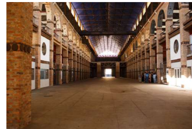
Fig. 149 Interior of the building. Photo by Mariana Leite, 2025. Source IPHAN
