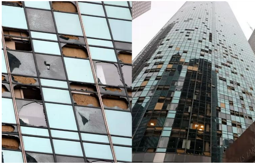
Figure 2- 24. Glass façade damage on a Houston high-rise.
