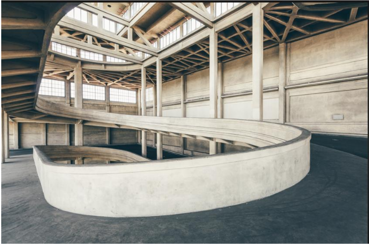
Fig81- concrete access ramps
