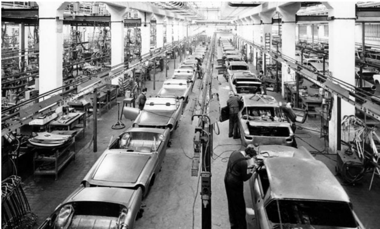
Fig.1 This is an image of part of the production line inside the Officine Stampaggi Industriali (OSI) factory. You can see the partially constructed Innocenti 950 Spyder on the left and the Fiat 2300 Coupes on the right.
