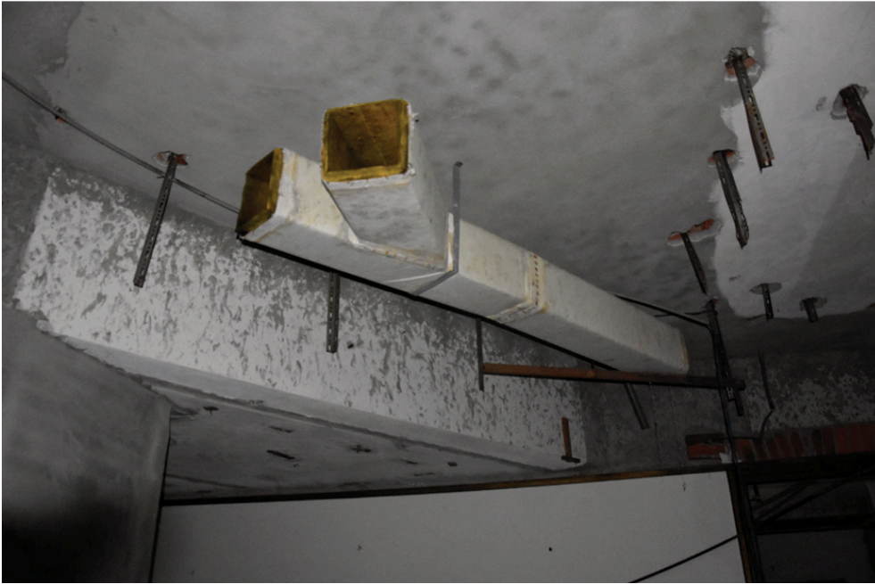
Picture 60. Supporting structure and channel for exposed ventilation.Archived documents
