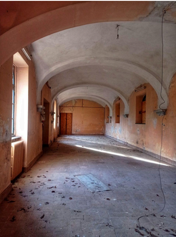
Picture 82 . Internal view of the system vaulted with arches of the sleeve east.Archived documents
