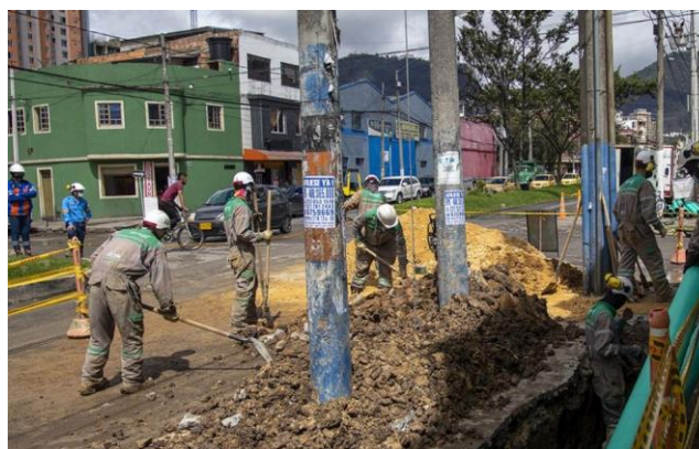
Figure 12 Underground network channeling using recycled aggregates.
