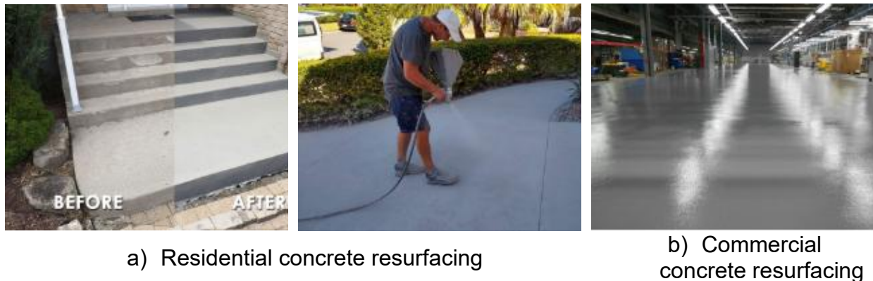
Figure 20. Concrete resurfacing [38]
