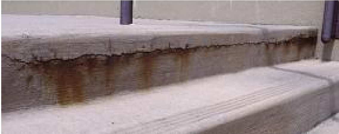
Figure 14. Corrosion Cracks
