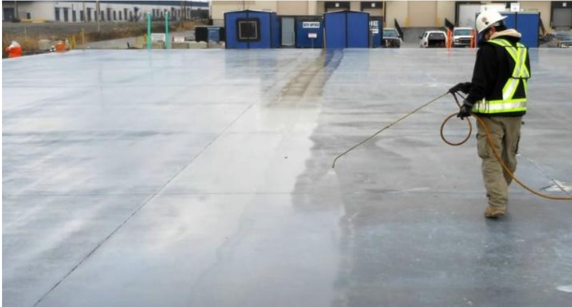
Figure 7. Spray curing concrete slab [24]
