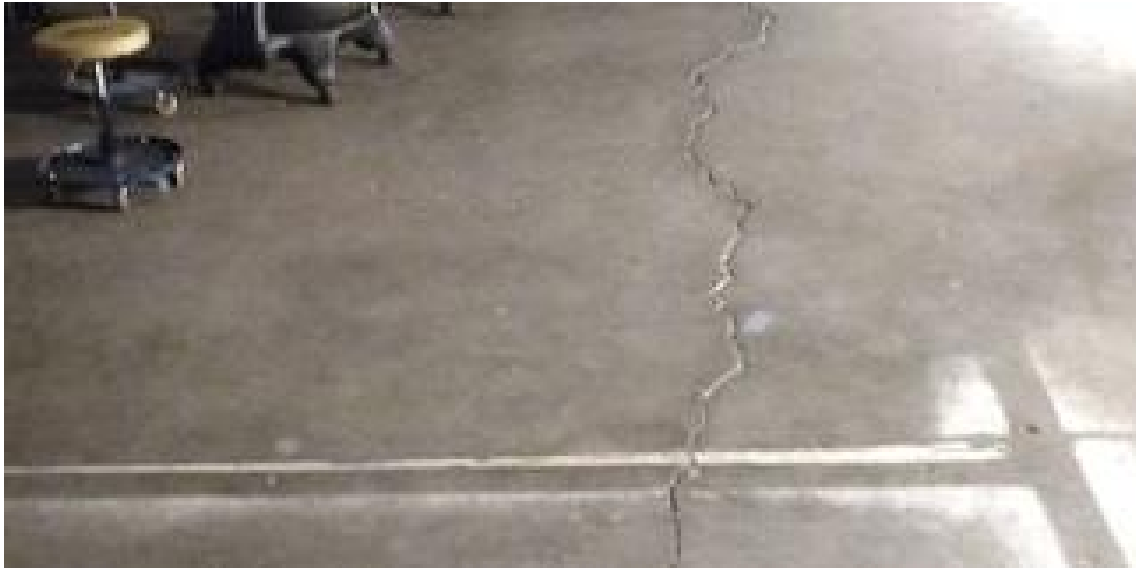
Figure 12. Long-term drying shrinkage cracks
