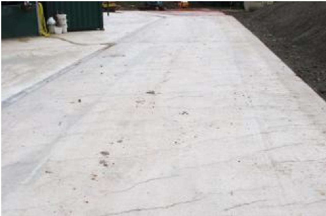
Figure 10. Plastic shrinkage cracks
