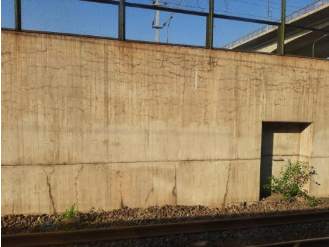
Figure 1. Example of thermal crack [4]
