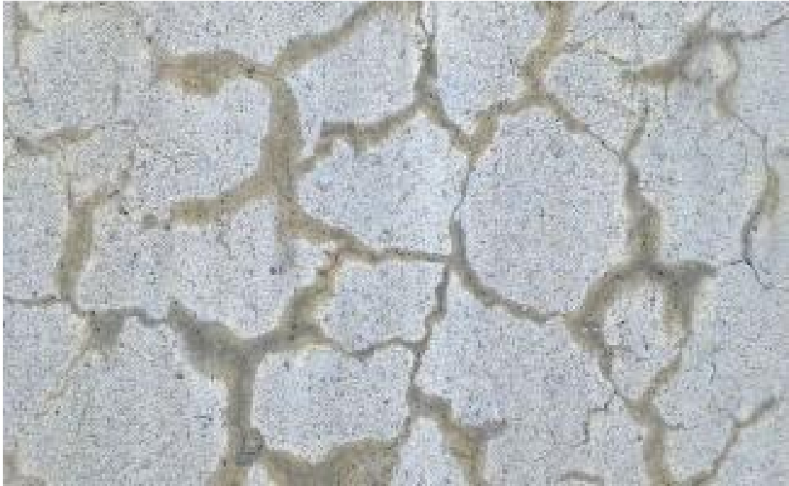
Figure 16. ASR and late expansion cracks [34]
