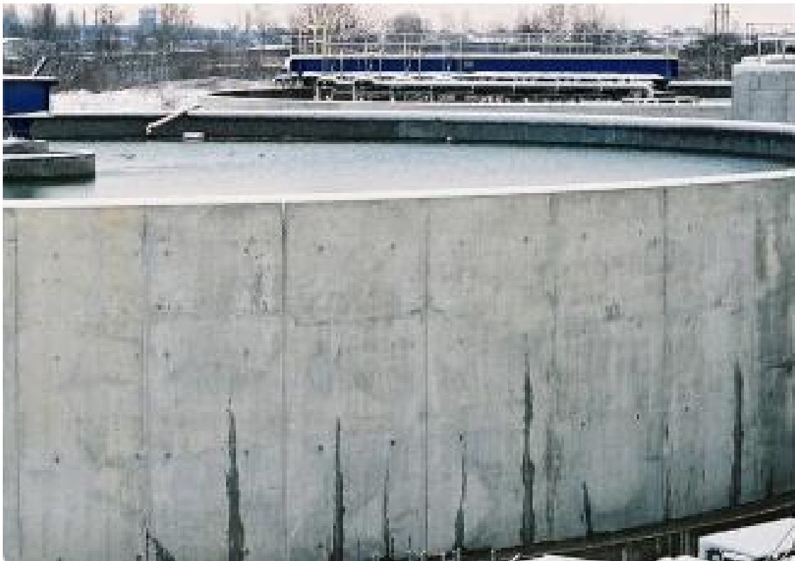
Figure 12. Long-term drying shrinkage cracks
