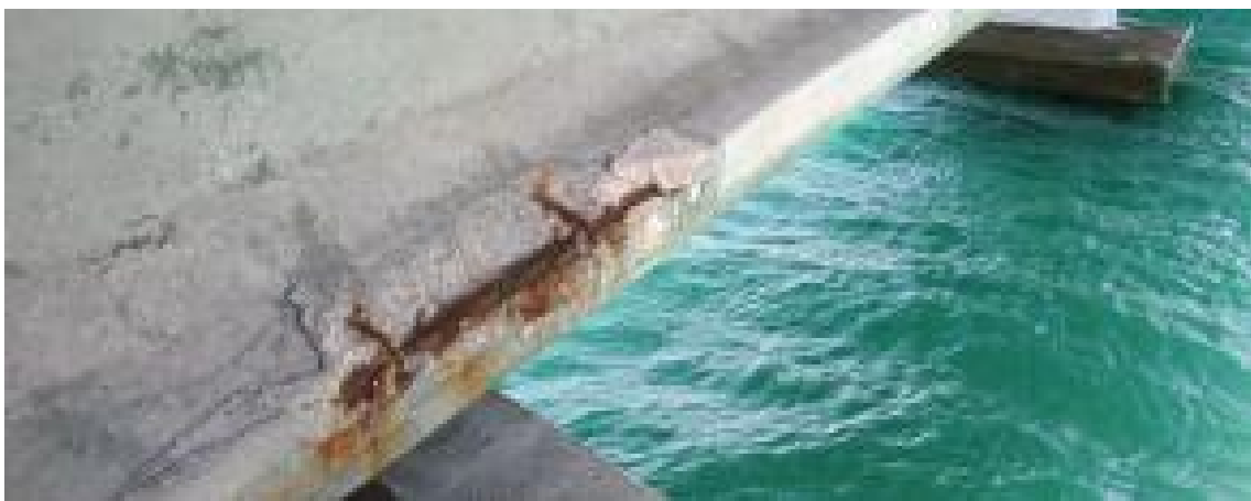
Figure 15. Corrosion Cracks
