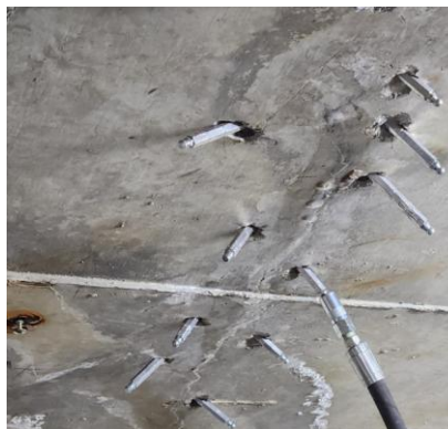
Figure 18. Concrete crack injection [36]
