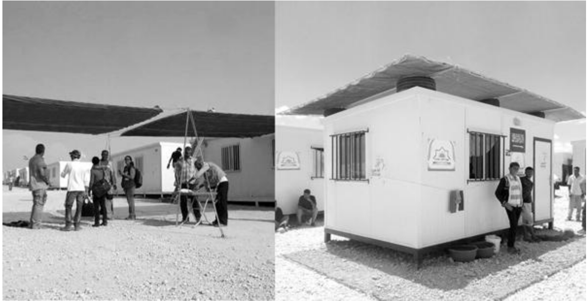
Shade roof and veranda. Prototypes of the kits made in Zaatari by an UNHCR implementing partner
