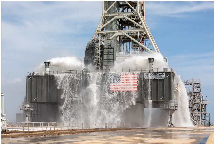
Figure 3.2: Kennedy Space Center's Sound Suppression Water System. -from NASASpaceFlight.com
