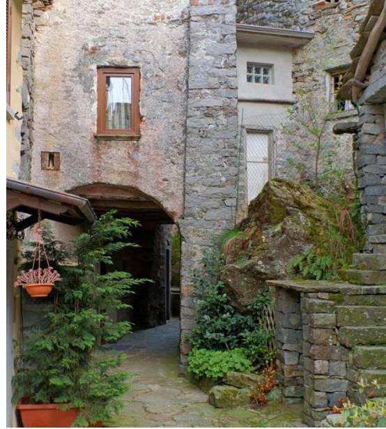
Figure 23 the stone row houses
