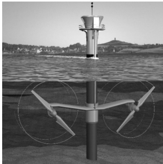
Figure 1.2-5: Seagen S-1.2 MW monopile tidal turbine [9]
