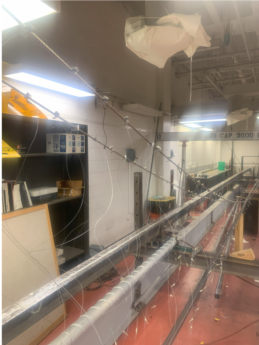
Figure 6.16: Hanger positioned at the correct distance.
