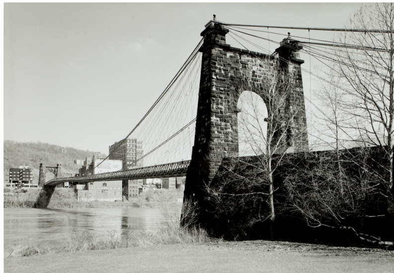
Figure 2.16: Wheeling suspension bridge rebuilt by John Roebling https://sah-archipedia.org/buildings/WV-01-WH22
