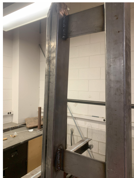
(b) Cross-beams of towers
