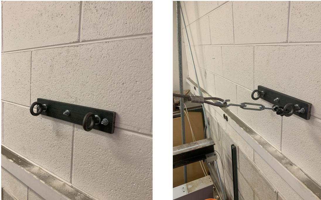
(a) Anchoring plate to the wall
