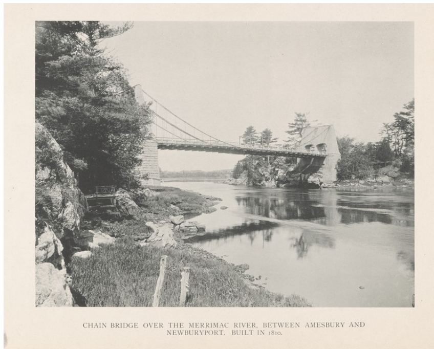
Figure 2.12: Chain Bridge over the Merrimac River, between Amesbury and Newburyport. Photograph from 1840. Digital Commonwealth.
