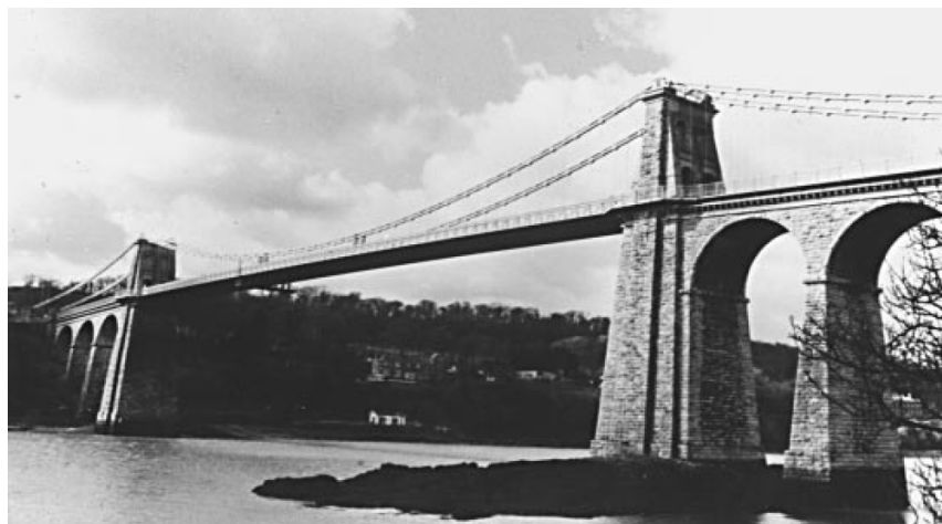
Figure 2.14: Menai Bridge in UK, in 1826
