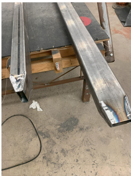
(a) Top of tower bended and welded
