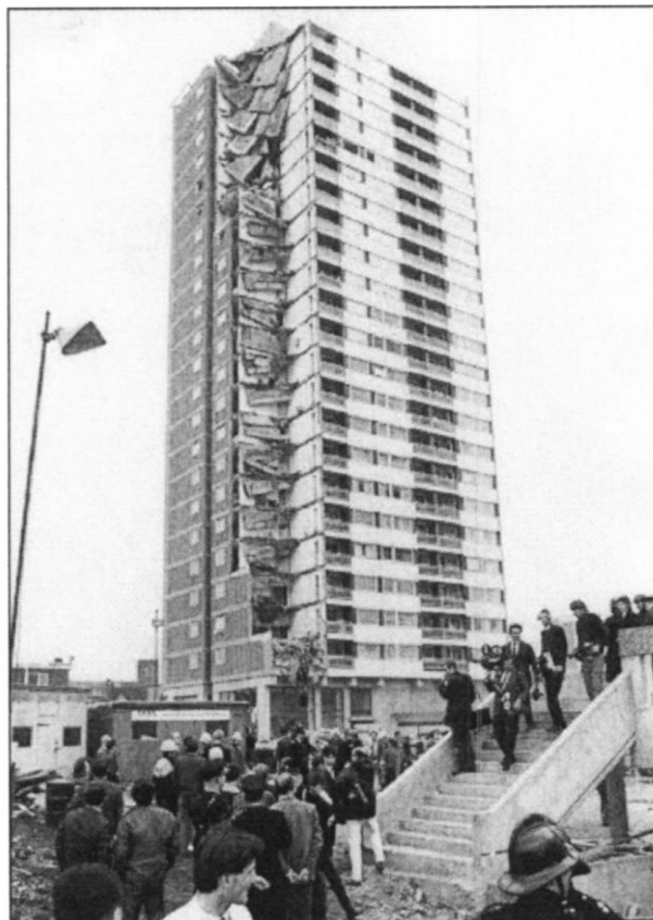
Figure 2.1 Ronan point building after collapse (Pearson and Delatte,2005)
