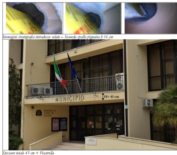
Figure 41-layers measurement_Ground Floor ceiling (END_S_03)
