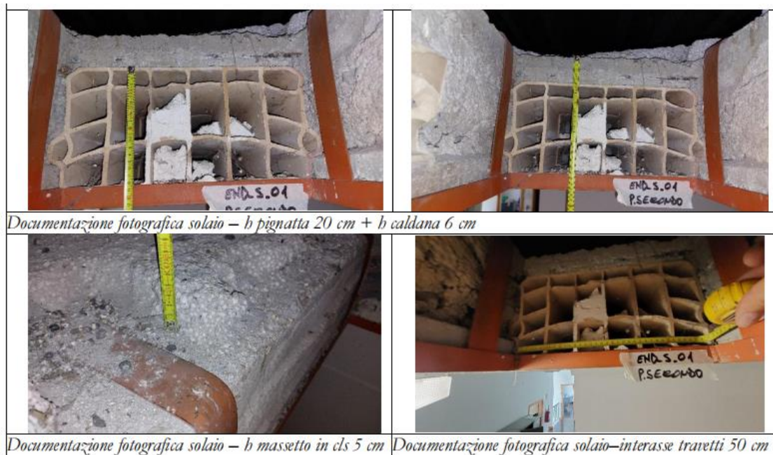
Figure 43-layers measurement _Second Floor ceiling (END_S_01)
