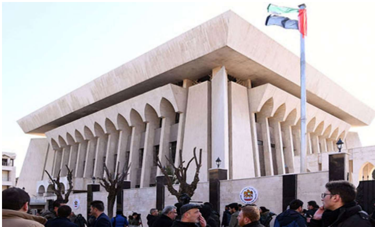
Figure 4.7 The embassy of the Arab Emirates, By SANA - arabnews.com
