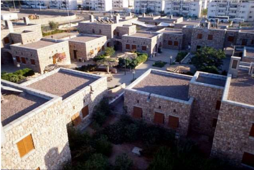
Figure 3.9 SOS Children's Village, Aqaba, Jordan (by arch. Jafar Tukan & Partners). Archnet
