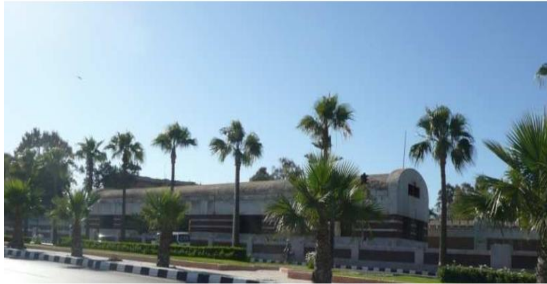
Fig.5.47. The parking lot of the Imperial Train of the late King Farouk, which is located beyond Montazah Castle. The structure is currently in a state of disrepair and is uninhabited. (Author)
