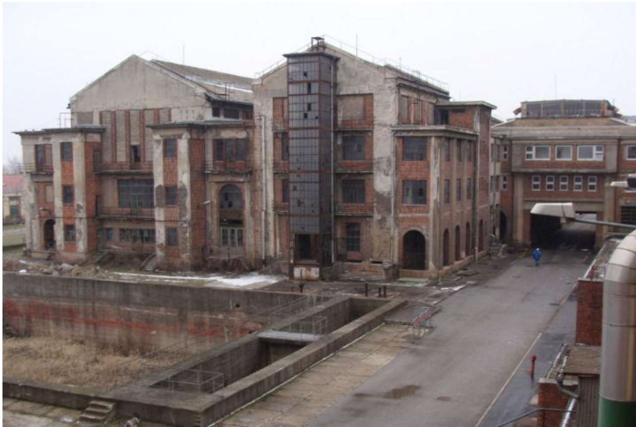
Fig.3.6. The disused Kelenföld Power Station located in Budapest, Hungary.
