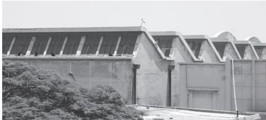
Fig.5.24. The new staining facility for fabrics of El-Shirka El-Ahliyya, 1960s expansion featuring north-facing sawtooth rooftop. (Alex Med)
