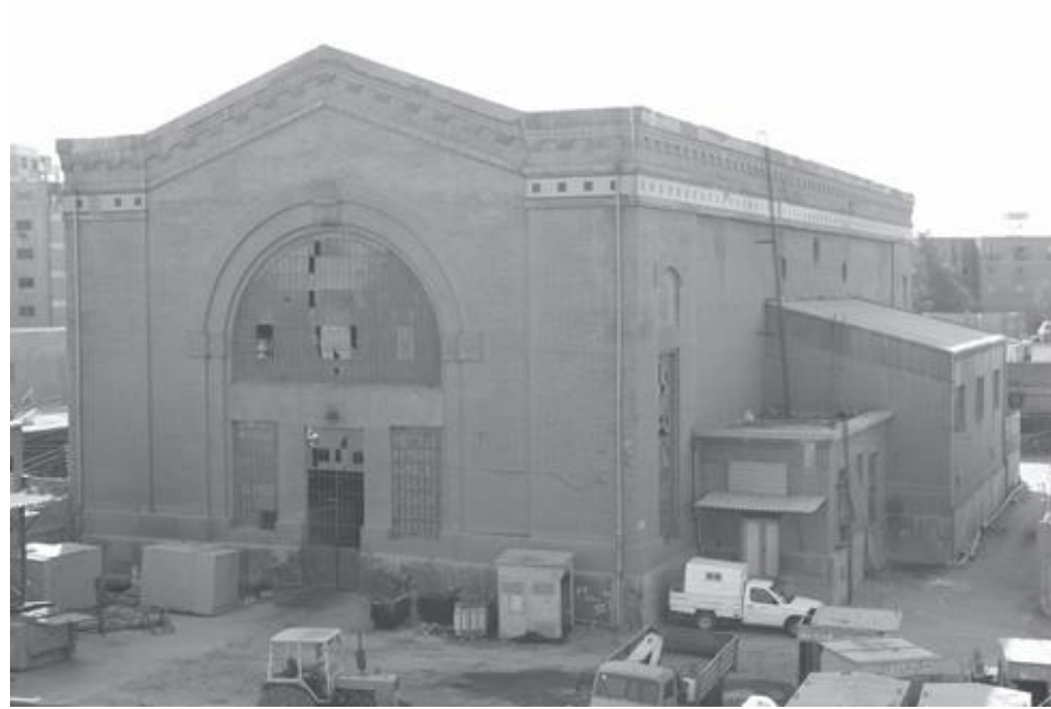
Fig.4.37. Tanta, Generator Building, 1931(The Alexandria and Mediterranean Research Center)
