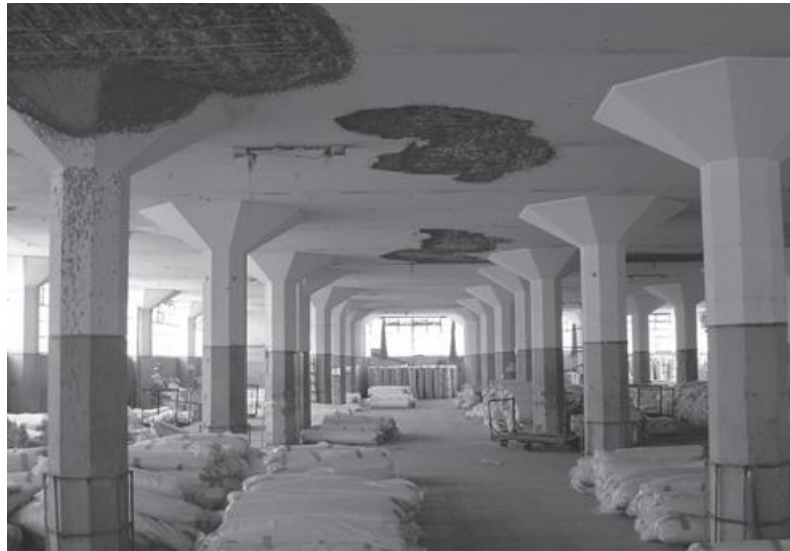
Fig.5.26. The wool plant operated by STIA, established by Ferdinand Debbané in the middle of 1950s; the inside shows mushroom pillars. (Alex Med)
