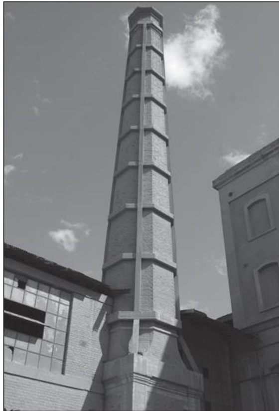
Fig.4.24. The concrete reinforcement that was later installed to the Salvago Ginning Plant smokestack
