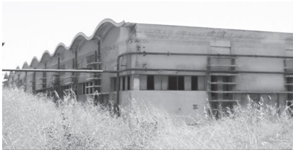
Fig.5.25. Al-Shirka al-Ahliyya, Expansions from 1962; perspective of the turbine edifice featuring a wavy multi-cylindrical shelled rooftop. (Alex Med)
