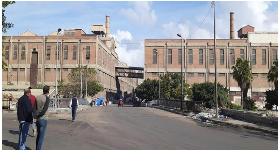
Fig.6.13. The bridge linking between the Nile and Masr presses. (Author & ANPIEMED)
