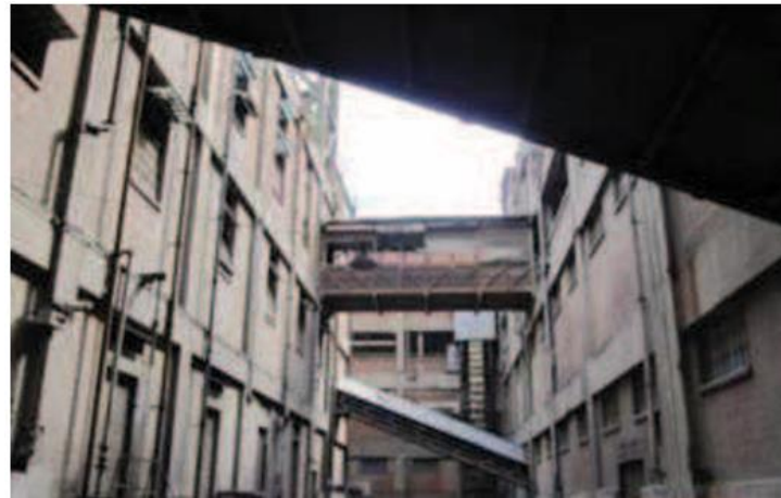
Fig.6.12. Current situation inside courtyard of Makbas El Nile (Author & ANPIEMED)
