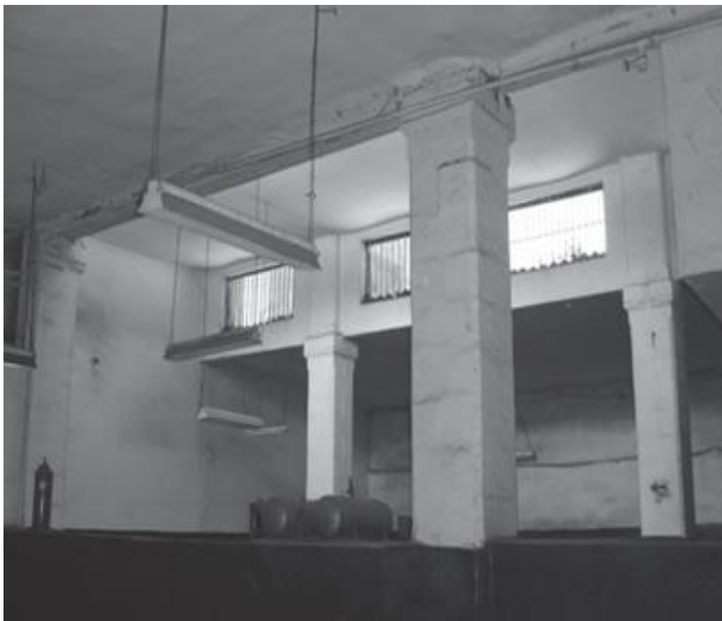
Fig.4.32. The interior expansion of the Spiro Spathis Soft-Drinks Manufacturing facility done in 1926, included stone pillars and a monitor ceiling. (Dar al wathaiq al- qaumiyyah. DWQ)
