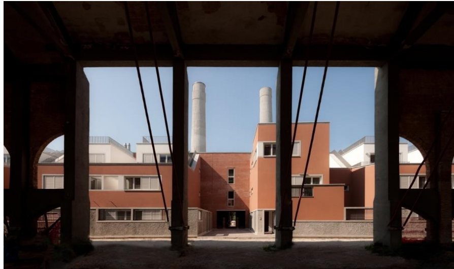
Fig.3.22. Studio Macola in Venice Italy which is renovated residential edifice.
