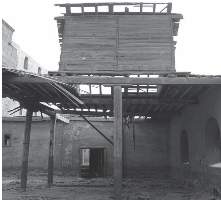
Fig.4.3. The workshop space adjacent to the cannon foundry at the Fortress Arsenal, showing the wooden ceiling adorned with a malqaf.
