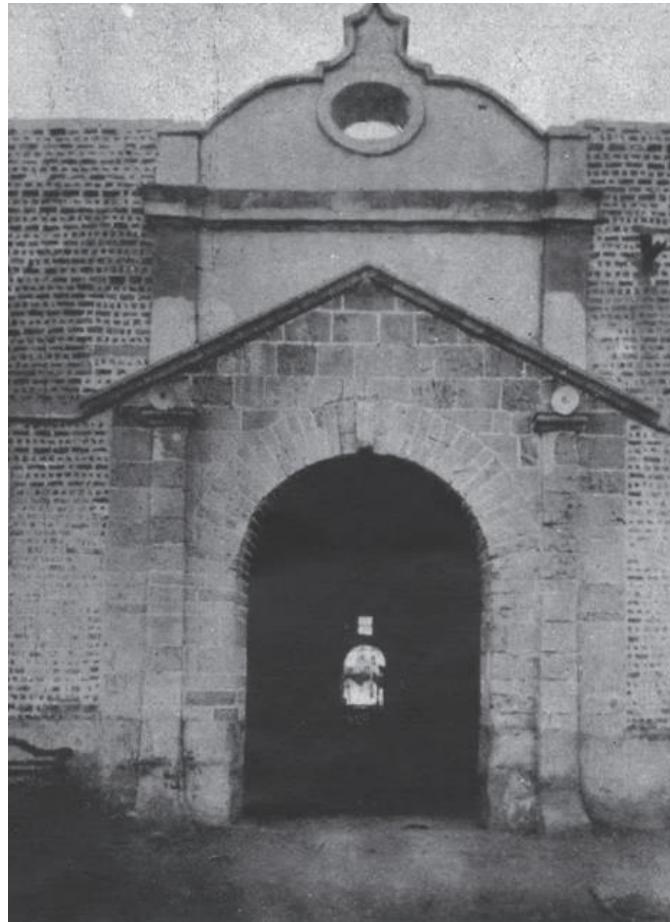
Fig.4.9. The entrance to a textile enterprise in Rosetta, dating back to the Mohammed Aly era, in 1820s or 1830s.
