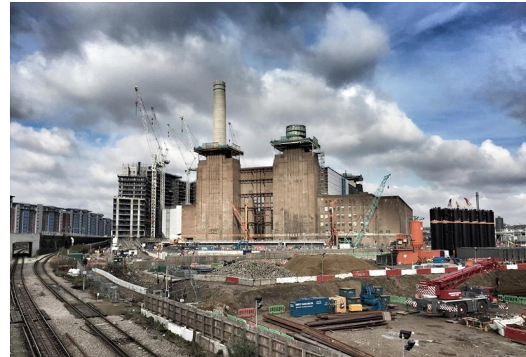
Fig.7.59. Battersea power station's chimney being removed 2016
