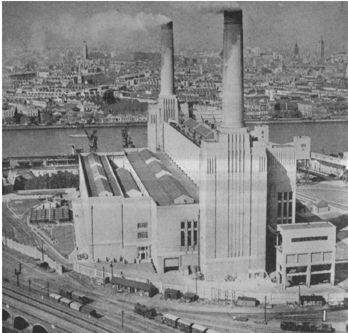
Fig.7.56. Battersea power station was built in two phases. This the first phase operational in 1934.
