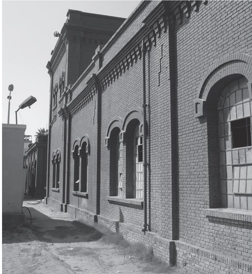
Fig.4.34. A perspective of the western façade of the filtration and pumping station, Tanta, Water Treatment Plants, 1926. (The Alexandria and Mediterranean Research Center)
