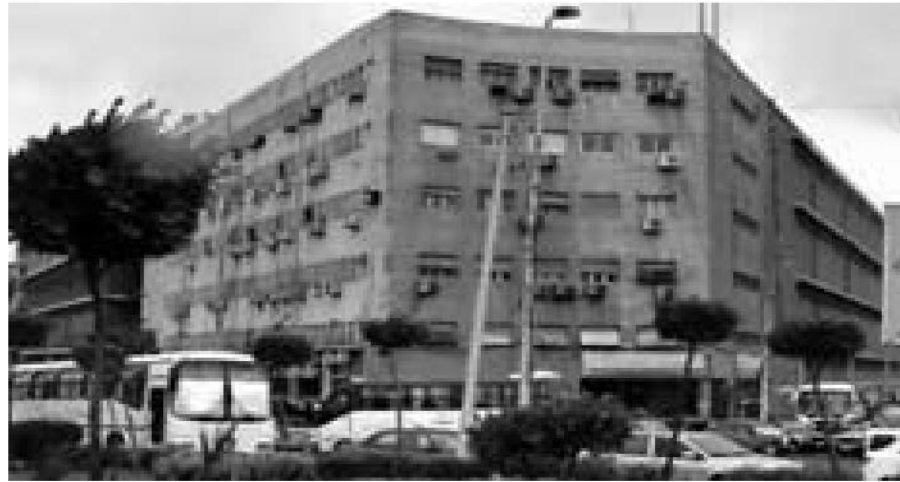
Fig.6.23. Bank of Alexandria, Mina El Bassal branch (Archives CEAlex)
