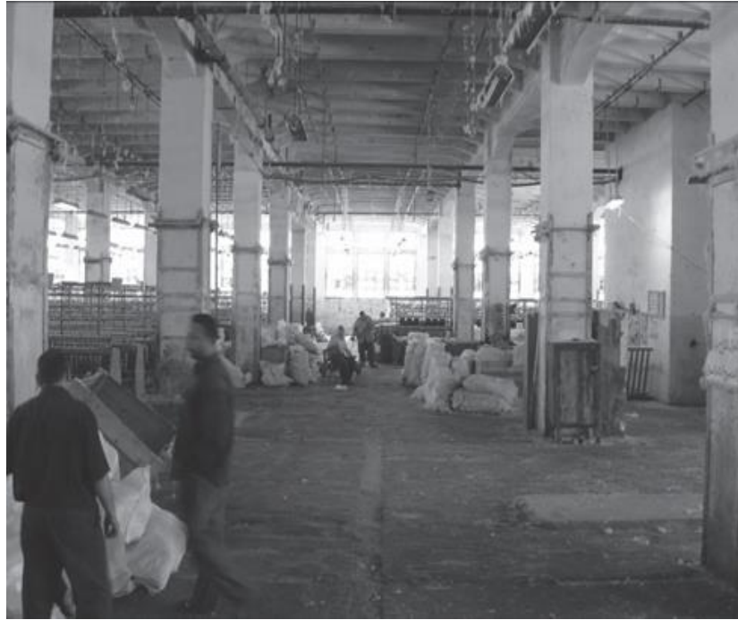
Fig.5.19. Internal perspective of the industrial hall of the novel structure of the Filature National d'Égypte.
