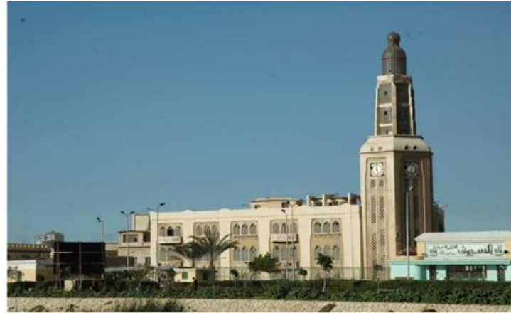
Fig.5.15. El Siouf Fabric Enterprise administration structure, which was once the Sepahi Factory. As emerging Islamic design gained popularity by that time, industrial construction began also to include architectural elements of such design. (The Alexandria and Mediterranean Research Center)
