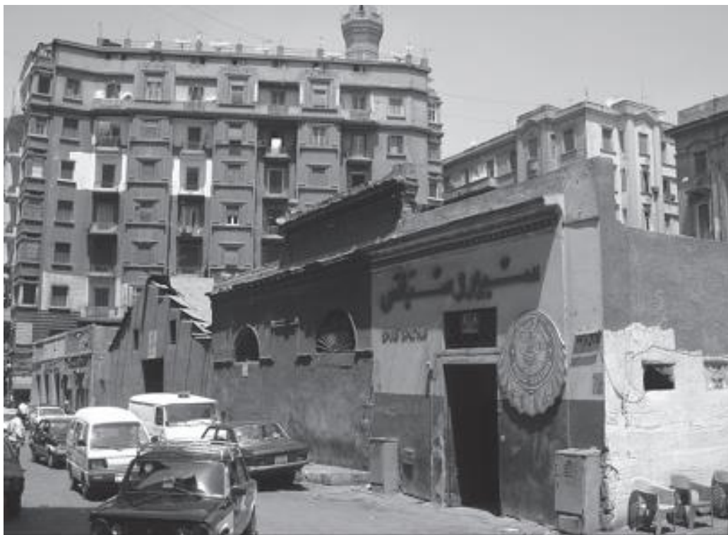
Fig.4.31. A perspective of the road's frontage of Spiro Spathis Fizzy Beverages Factory in Bab El-Hadid Area, Cairo, during the first decade of the 20th century. (Dar al wathaiq al- qaumiyyah. DWQ)
