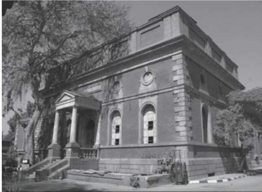
Fig.4.29. Giza, Waterworks, pump house, 1896. (Dar al wathaiq al- qaumiyyah. DWQ)
