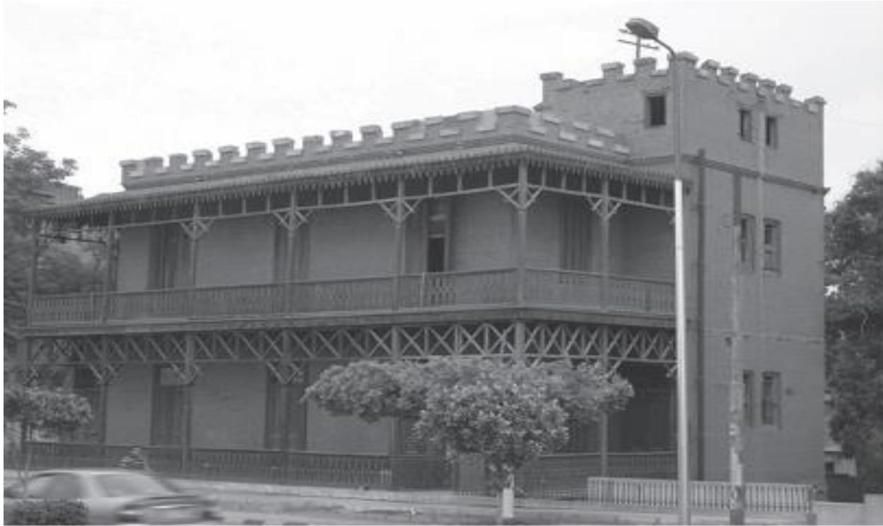
Fig.4.19. Salvago Ginning Mill, guesthouse, after 1895. (The Alexandria and Mediterranean Research Center)
