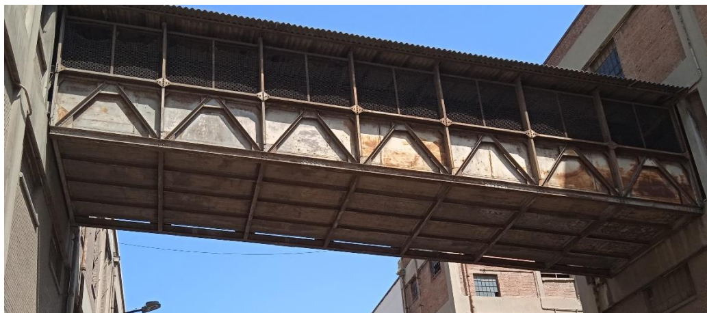
Fig.6.14. The bridge linking between the Nile and Masr presses. (Author & ANPIEMED)
