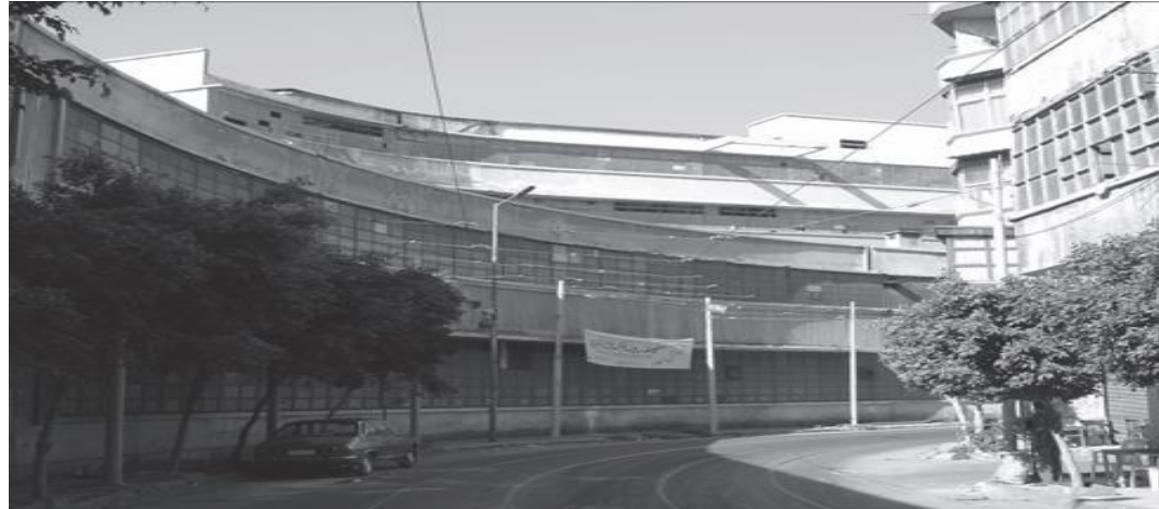
Fig.5.28. STIA operates, road frontage perspective of the southern sections. (Alex Med)
