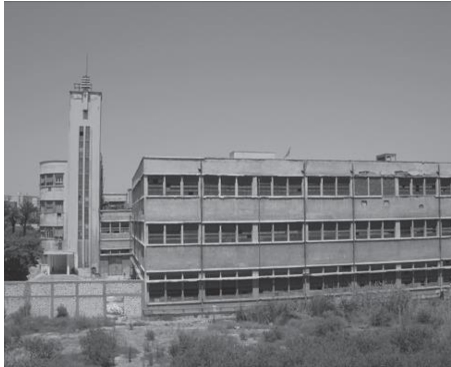
Fig.5.18. The newly constructed workplace of the Filature National d'Égypte, with the elevator shaft and the western industrial edifice.
