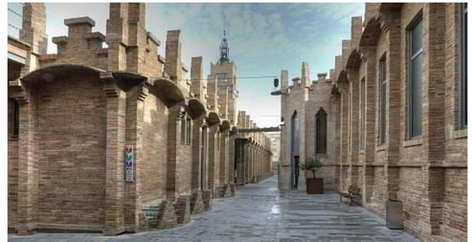
Fig.7.69. Caixa Forum in a former textile factory from the time of Modernism
