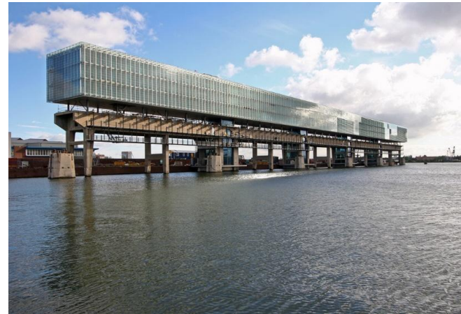
Fig.3.14. Skin intervention. Kraanspoor, meaning crane, is a lightweight, glass office structure with three levels, constructed on a concrete crane. Architects: OTH Architecten, 2007
