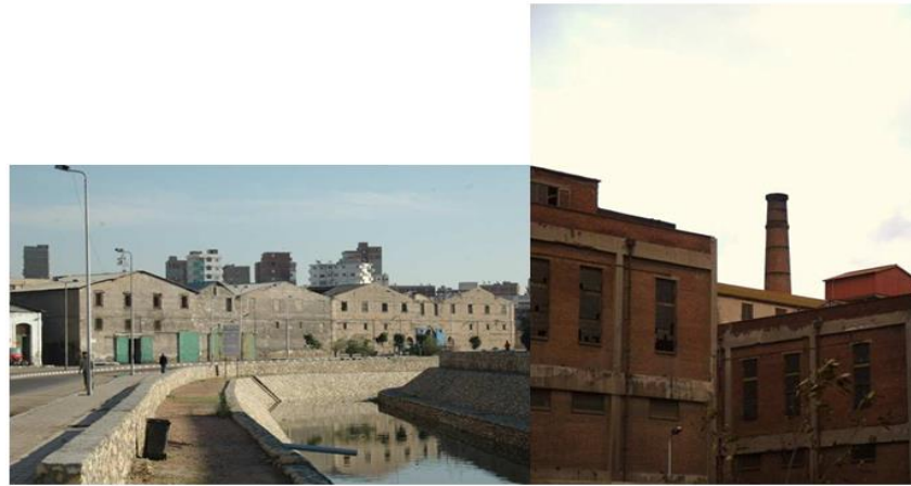
Fig.5.4. Two kinds of warehouses are seen, the left one with Supporting walls while the right one shows a concrete reinforcement frame featuring visible slabs of concrete and redbrick filling. (The Alexandria and Mediterranean Research Center, Bibliotheca Alexandrina)
