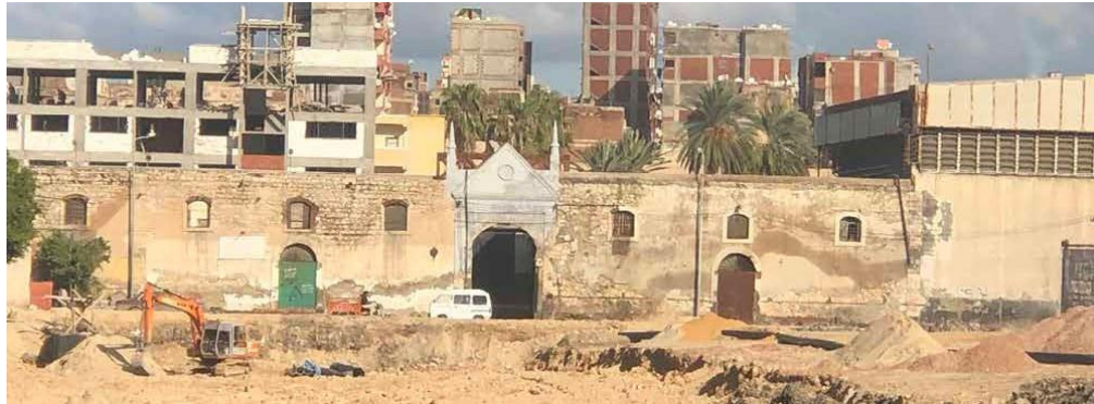
Fig.5.5. The Northeast perspective of the remaining upright eight thousands m 2 warehouse of Amin Bey, intended for cotton. (ANPIEMED)
