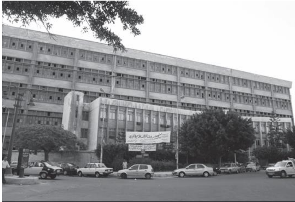
Fig.5.32. The novel wool facility of STIA company in Hadra District, Alexandria (Abu al-Fadl, Hadari, and Khuli in 1974); a perspective of the southern frontage of the administrative edifice and the central industrial complex oriented towards Sirri Pasha Square. (Alex Med)
