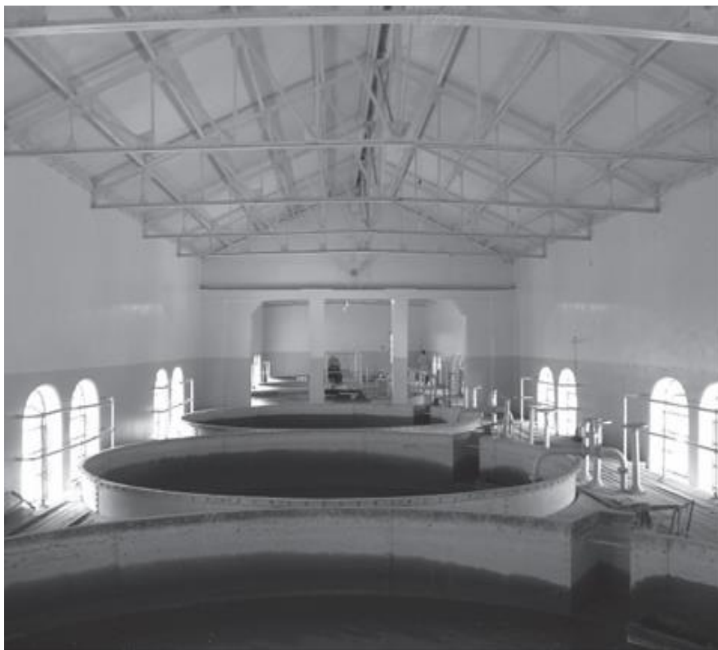
Fig.4.35. A perspective of the interior of the filtration and pumping station, Tanta, Water Treatment Plants.
