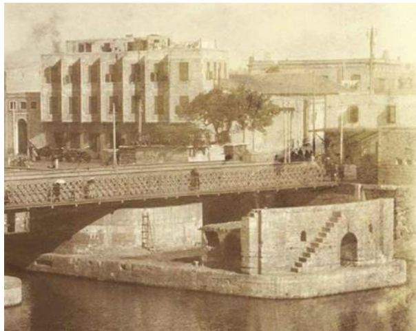
Fig.5.10. Storehouse Dahan is largely blended with Arab houses, distinguished by its angular, upwards projecting façade. The edifice overlooks the inaugural bridge linking both banks of the Canal. The bridge is known as Kobrī at-Tarīkh, (Late nineteenth century and early twentieth century. ( Dar Al-Watha'iq al-Qawmeia ))
