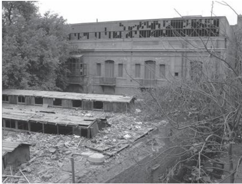
Fig.4.28. Railway Telegraph Stores, view of northern facade. (Dar al wathaiq al- qaumiyyah DWQ)
