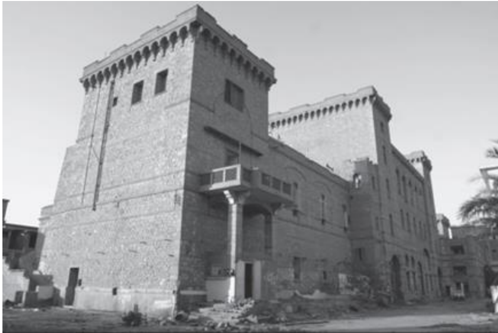
Fig.4.26. A perspective of the western extension and the core building of the Brasserie des Pyramides Brewery.
