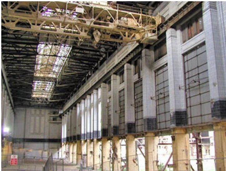
Fig.7.58. Station turbine hall 2006
