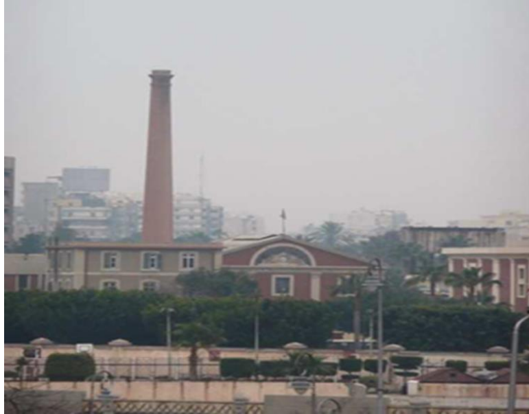
Fig.5.44. Constructed in 1886, the Alexandria Water The organization's smokestack and building are a beautiful addition to the cityscape of Alexandria. (Alex Med)
