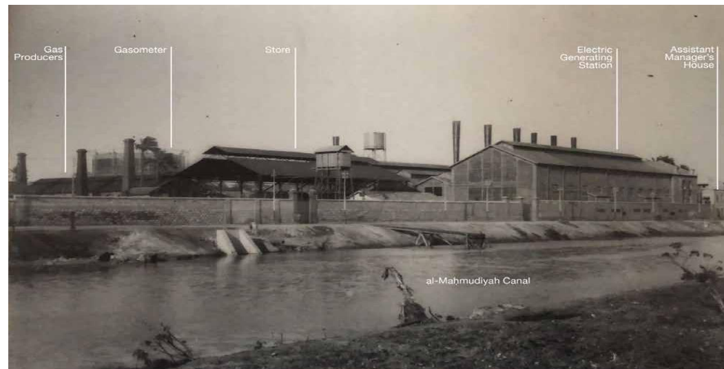
Fig.5.35. A picture illustrating the gaswork in Alexandria at the north shore of the canal and its different edifices (Archives CEAlex).
