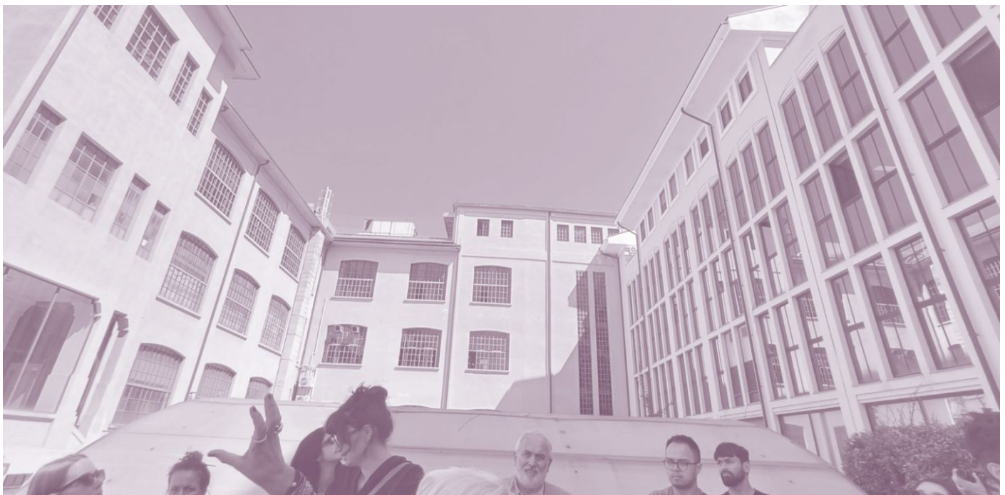
Fig. 45. Courtyard of the Ex-Borsalino Factory – currently a university residence and mixed-use complex. Building to the left was designed by Arnaldo Gardella in 1925, and to the right was designed by both Ignazio and Jacopo Gardella. Source: Author – Taken on June 27, 2024.
