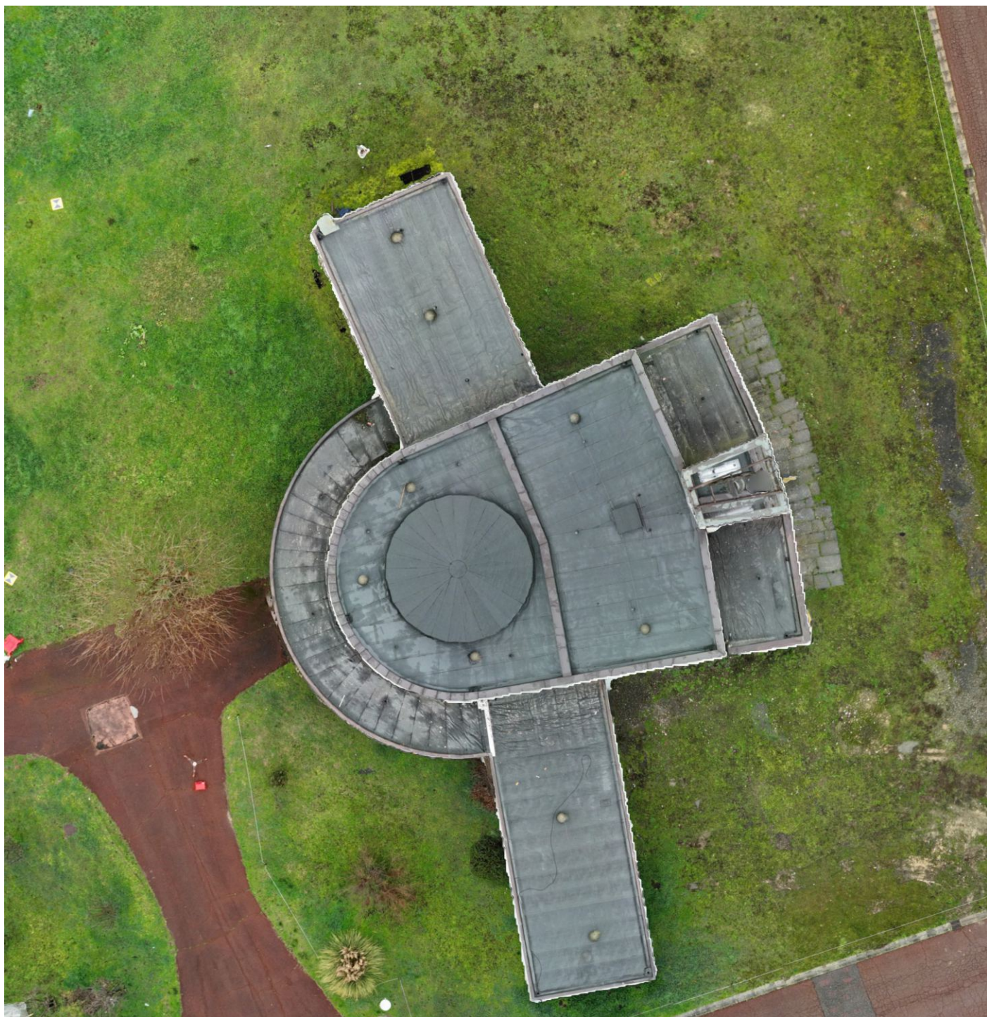
Fig. 56E. Roof View Orthophoto (Aerial Range Chunk).
