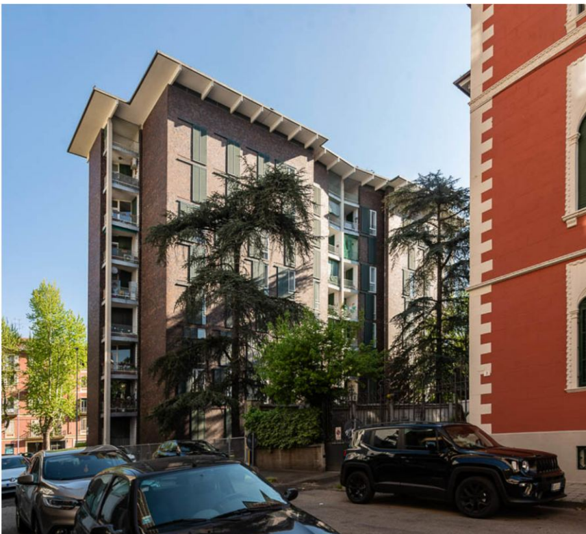
Fig. 55. South Façade view from Via Messina. Source: Flickr.com by Jacqueline Poggi – Taken on April 24, 2023.
