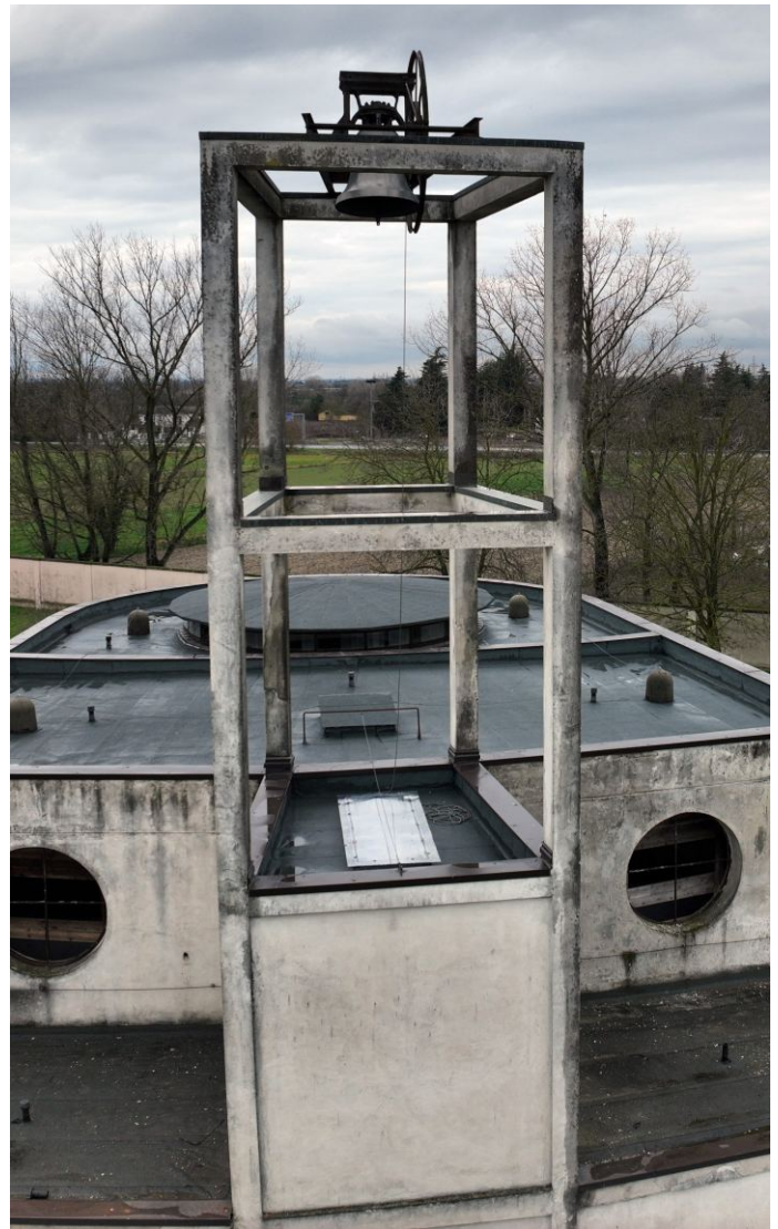
Fig. 8 (left). Perspective views of the Bell Tower, showing a column beam structure. Source: by the authors.
