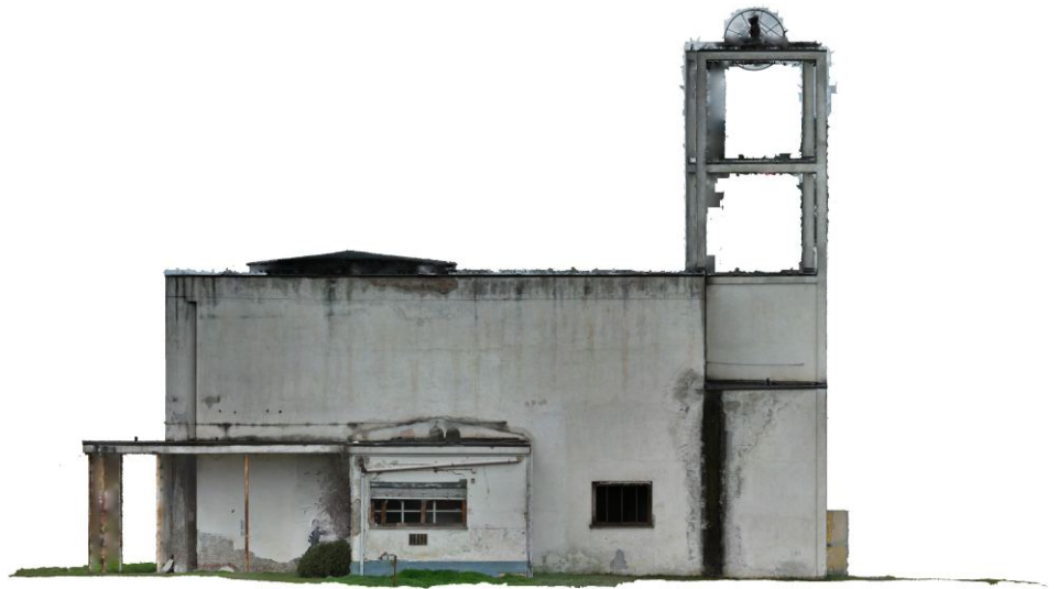
Fig. 56B. South Façade Orthophoto.
