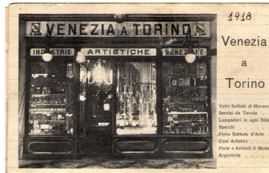
Figure 77 - Historical photograph of the facade of Venezia a Torino, possibly from 1918
