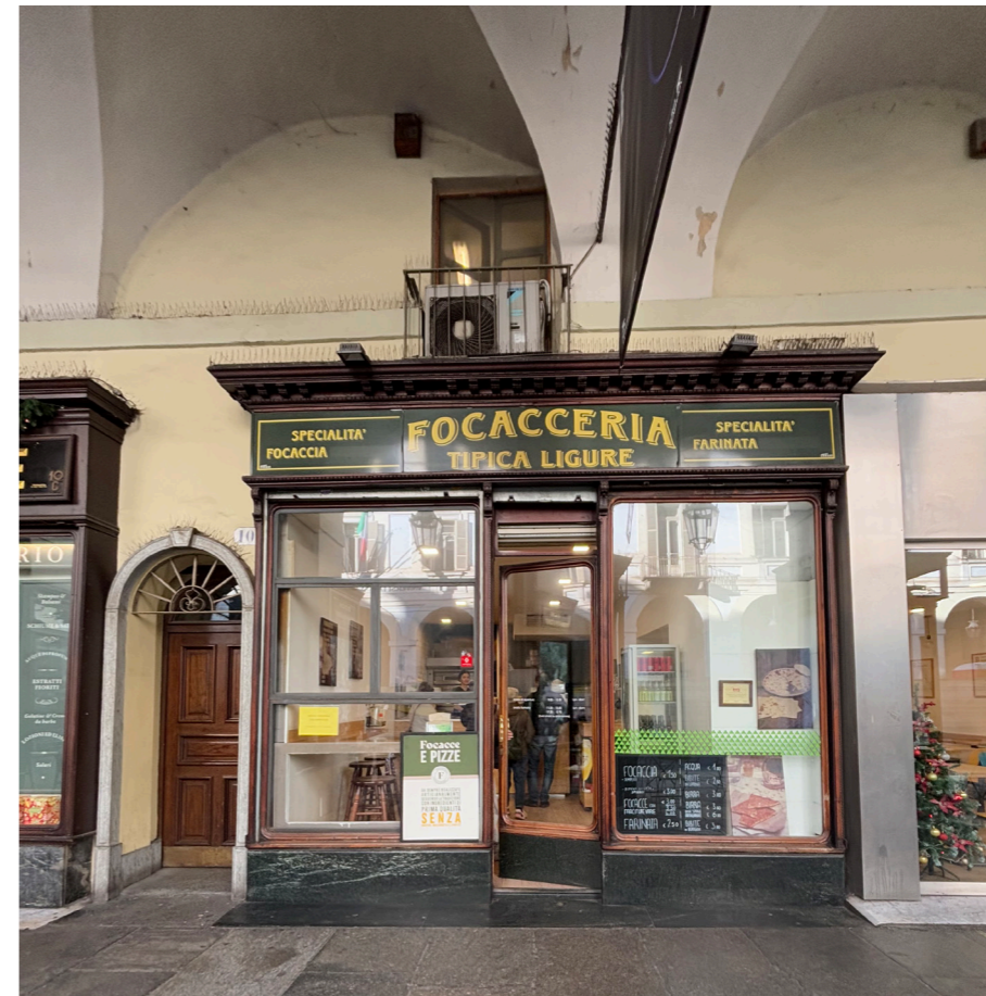
Figure 64 - Photograph of the facade of Focacceria Tipica Ligure, ex-Reale Ombrelleria Artigiana
