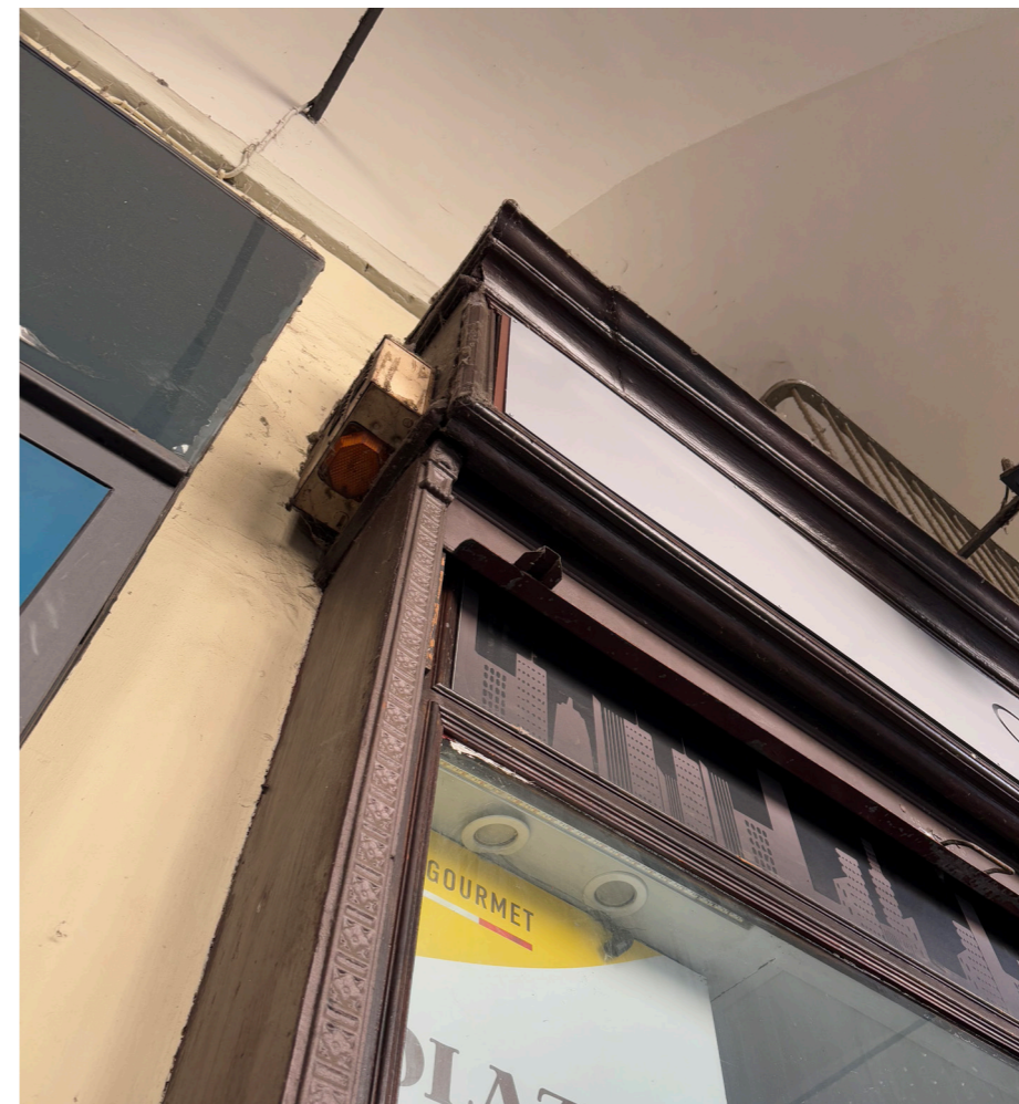
Figure 95 - Detail photograph of the wooden frames of the monoblock and the sign box of the facade of the shop space 1
