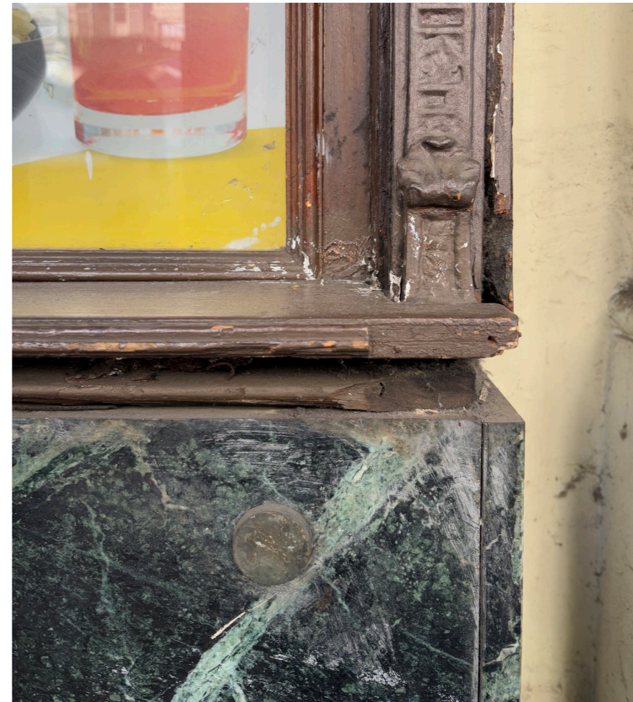
Figure 94 - Detail photograph of the green marble plinth and the wooden frames of the monoblock of the facade of the shop space 1
