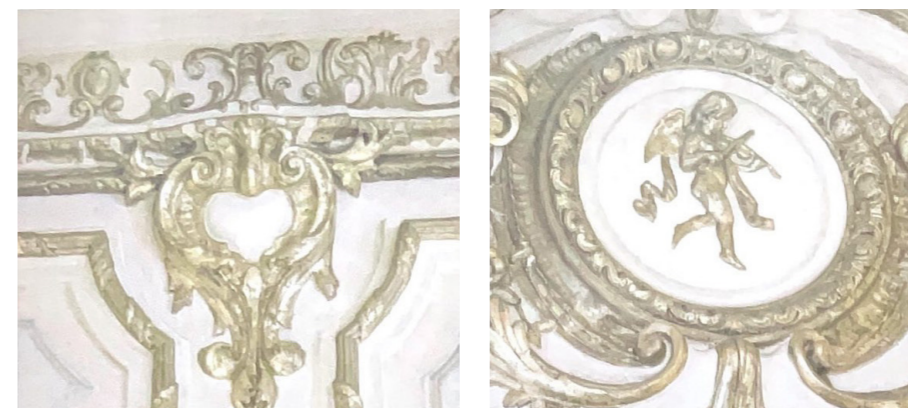
Figures 12-13 - Detail photograph of the interior decoration in gilded stucco of Liquoreria Confetteria Caffè Platti
