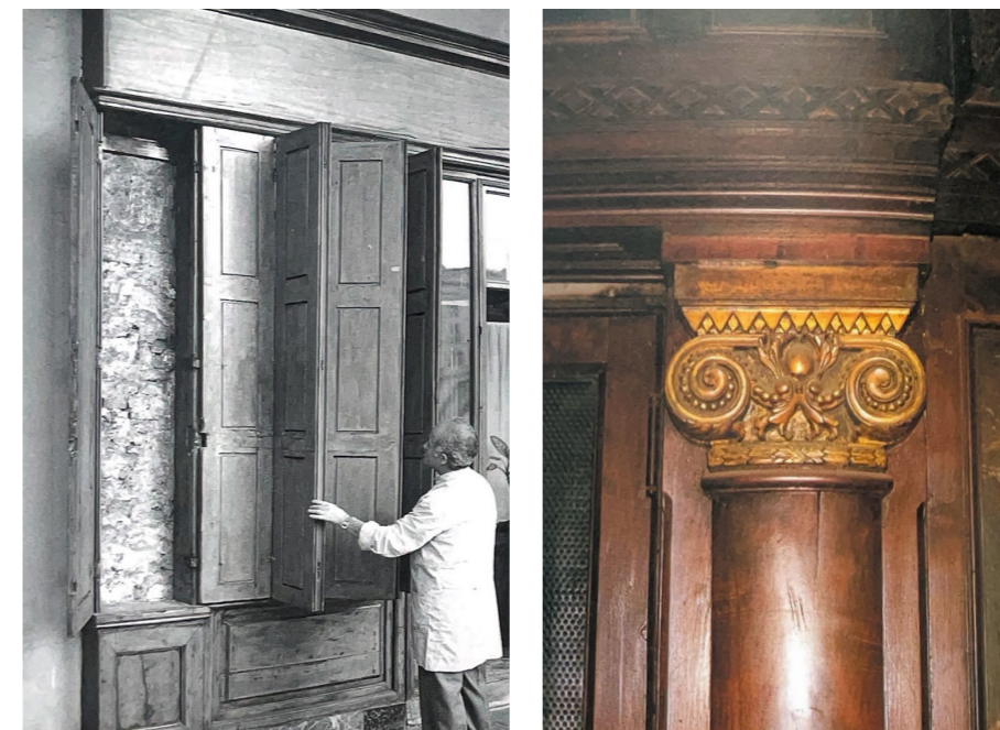
Figure 49 (left) - Detail photograph of an example of wooden shutters used in a barber shop in Piazza Vittorio Veneto
