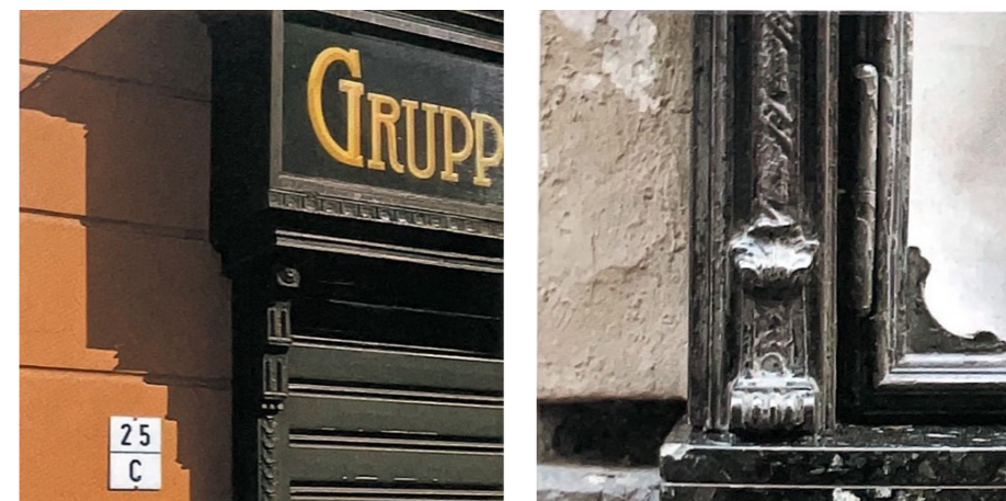
Figures 52-55 - Compilation of detail photographs of the application of iron on facades of historic shops
