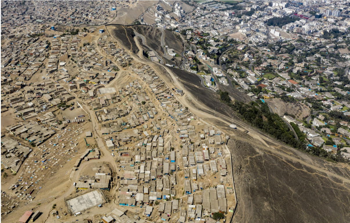
Figure 39: Neighborhood of Pamplona Alta (informal city) and Neighborhood of Surco (formal city), Lima.
