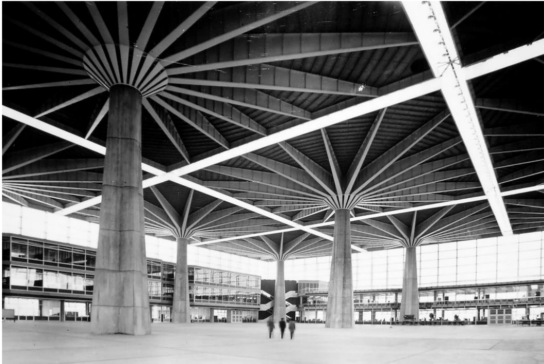
Figure 59 Palazzo del Lavoro, Mushroom columns and the internal space.
