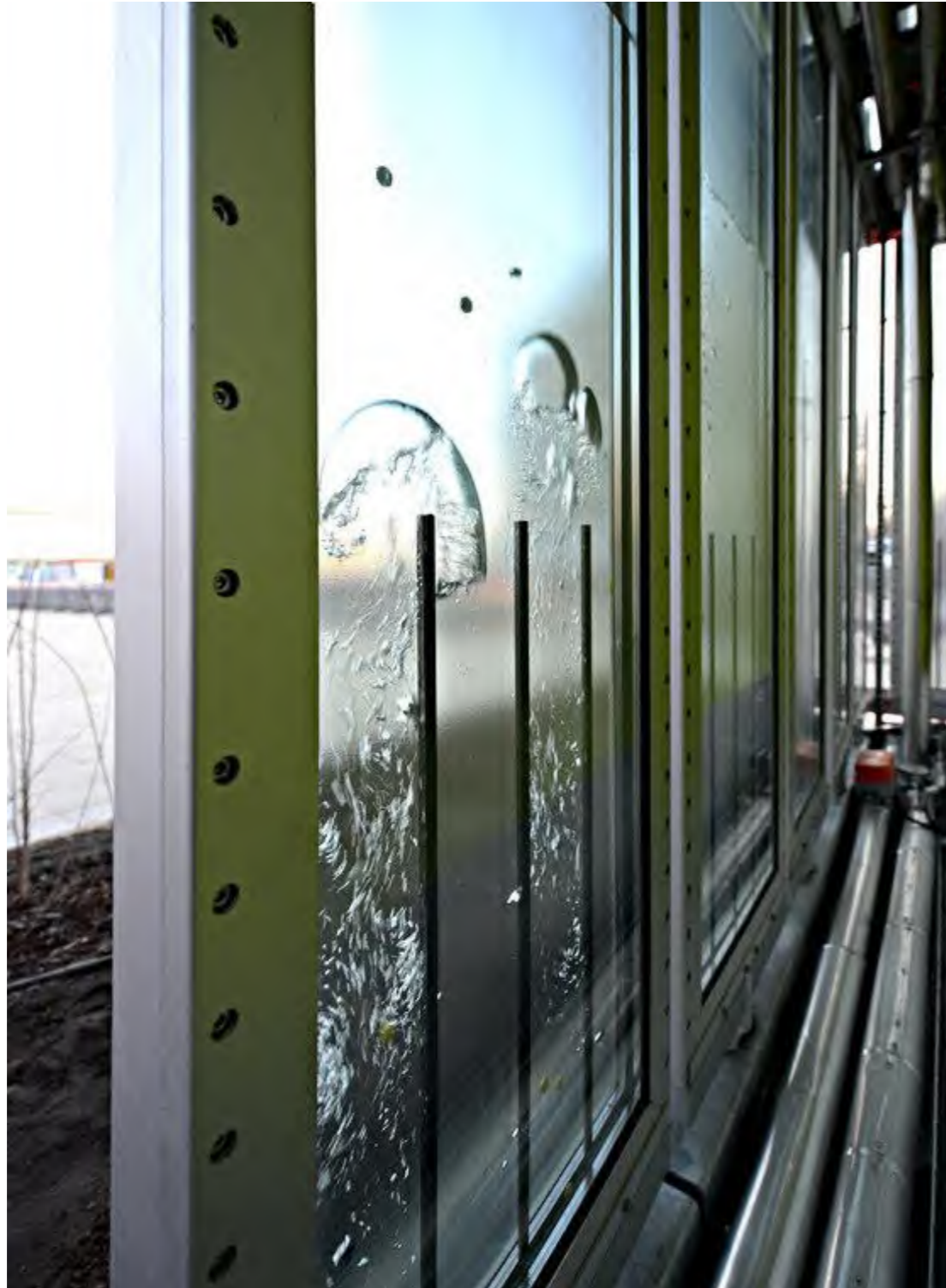
Figure 7 : Solar Leaf - The World's first Algae-biomass producing Facade System [Photograph]; Solar Leaf-Louver viewed from Backside with hidden Horizontal Support System. courtesy arup/splitterwerk. (2013). Retrieved from https://www.designboom.com/art/worlds-first-algae-powered-building-by-splitterwerk/
