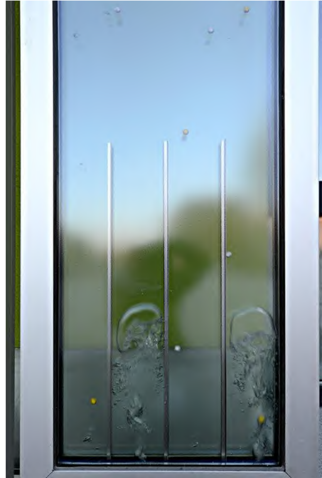
Figure 5 : "SolarLeaf - The World's first algae-biomass producing facade system [Photograph], courtesy arup/splitterwerk. (2013). Retrieved from https://www.designboom.com/art/worlds-first-algae-powered-building-by-splitterwerk/
