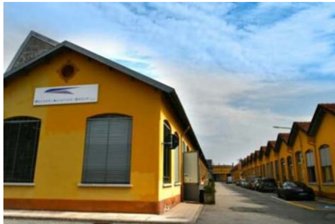
Figure 2: View of Borgomanero factory
