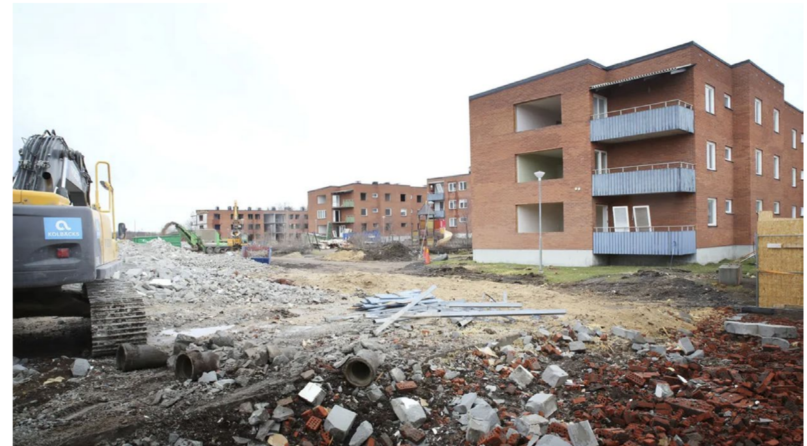
Demolition of Ullspiran. From TU.
