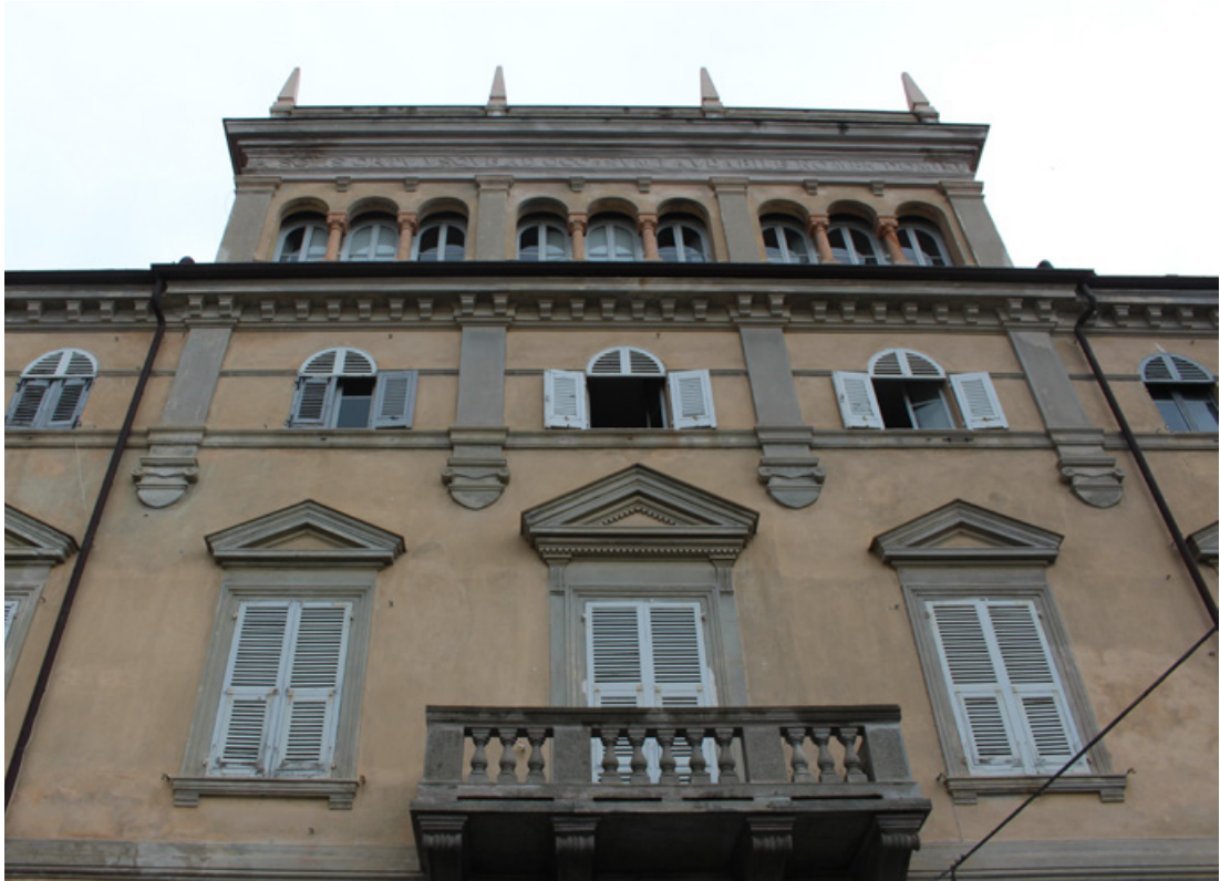
Figure 16. Balcony, windows and triangular pediments.
