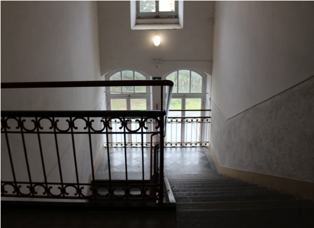
Figure 27. One of the internal stairs.
