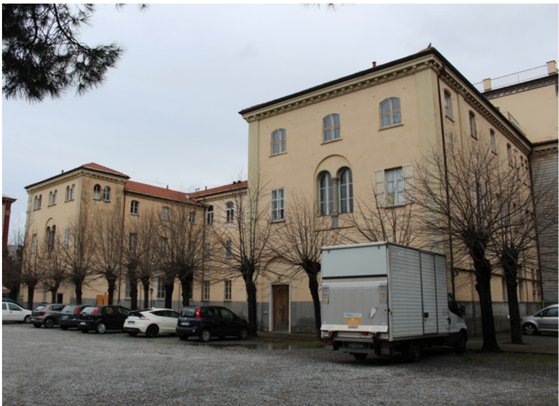
Figure 17. The east facade, with its half-open courtyard.
