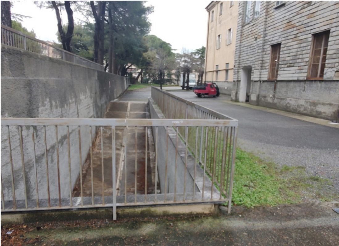
Figure 11. Driveway ramp (photo by Lorenzo Savio).
