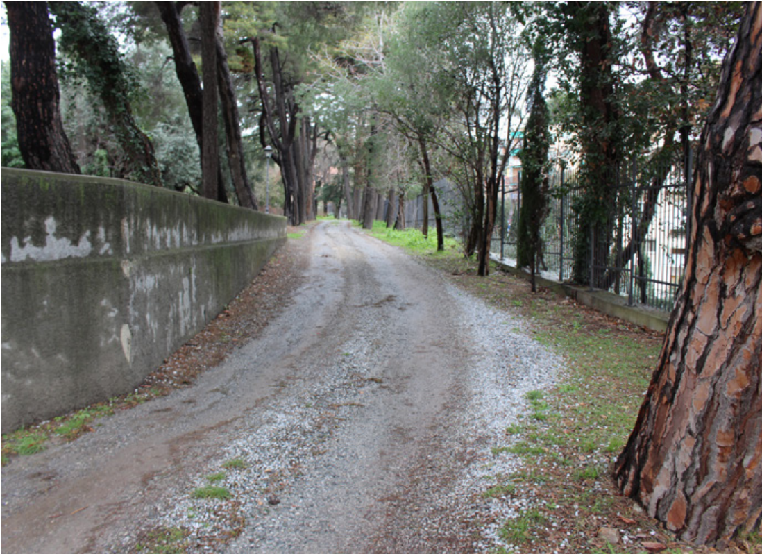
Figure 10. Driveway and garden retaining wall.
