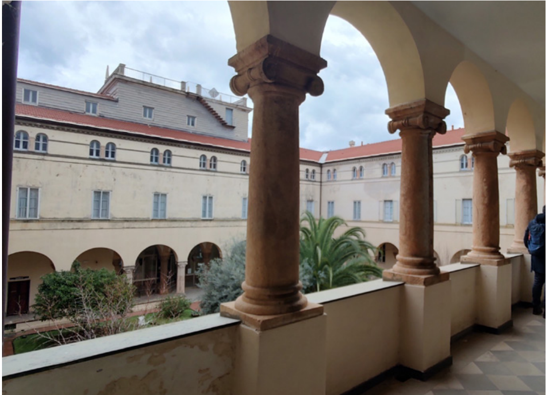
Figure 33. View from the portico at the first floor (photo by Lorenzo Savio).
