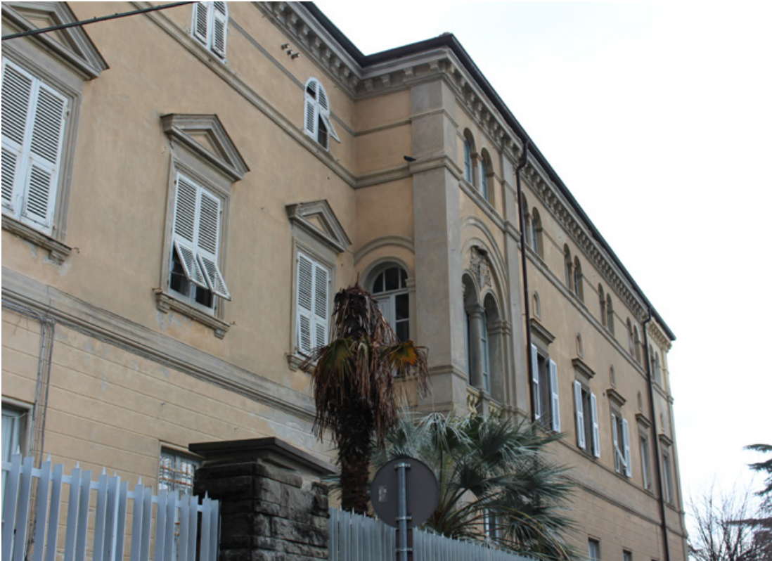
Figure 15. Second floor openings.
