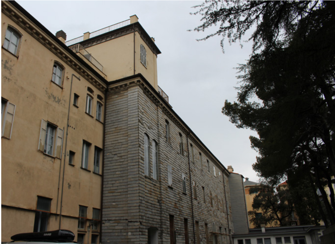
Figure 18. The rear facade, covered with a typical technique known as ardesia inchiappata .
