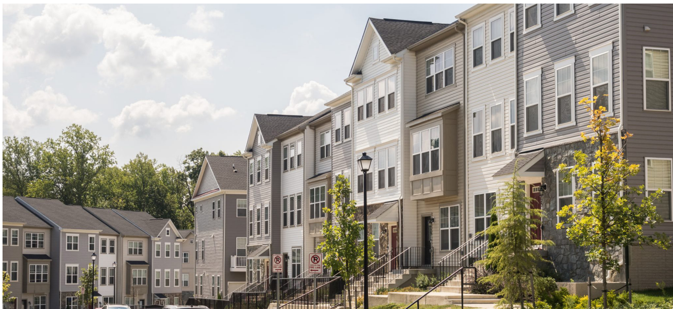
Image 1: Affordable houses project in Montgomery County - (Montgomery, n.d., "Affordable Housing")
