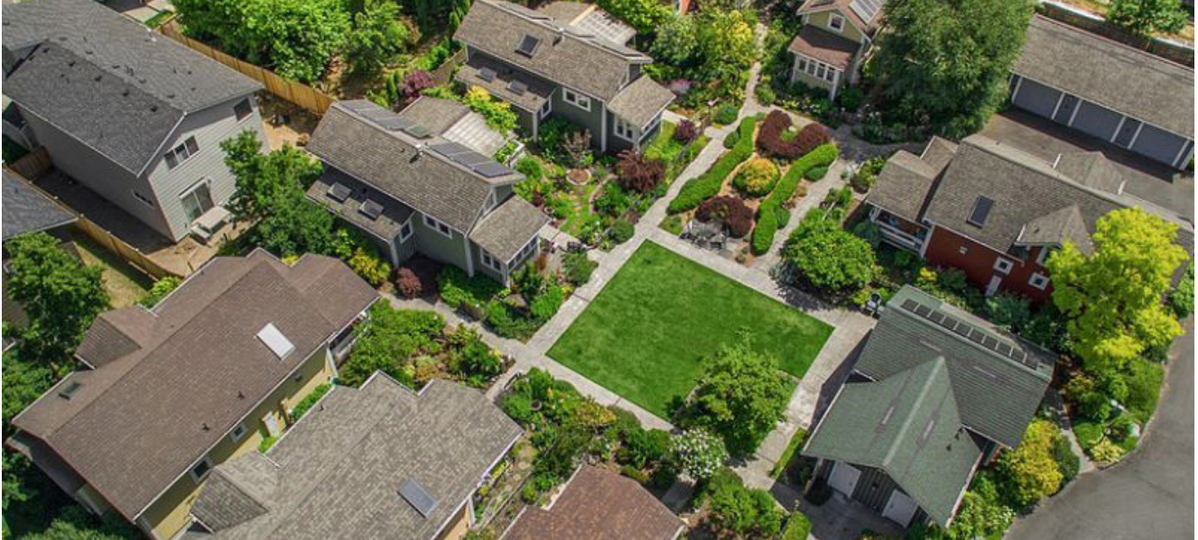
Image 1: Aerial view of Cottages project - (Chapin, n.d., "Greenwood Avenue Cottages")
