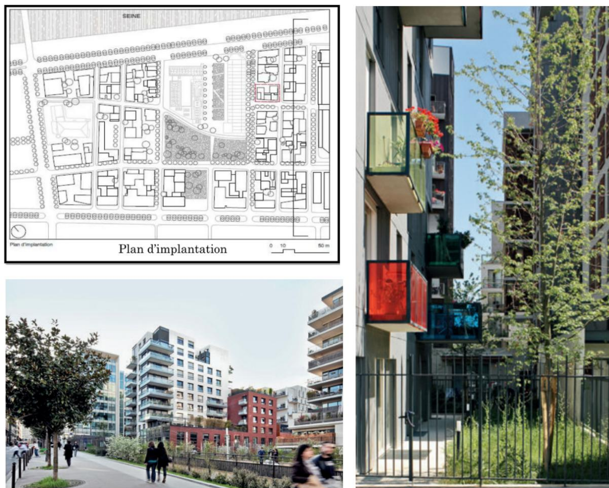
Fig 3-10 General plan and pictures of development in the Massna - Grands Moulins area on the left bank of the Seine, Paris (source: Friedberg, 2019)
