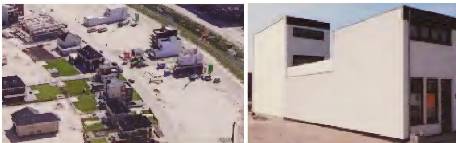
Fig 4-11 Housing type in Almere Poort community in the Netherlands (source: archdaily)
