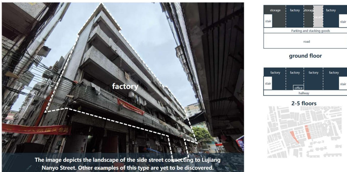
Fig 2-19 Production space adjacent to secondary streets (source: the author)
