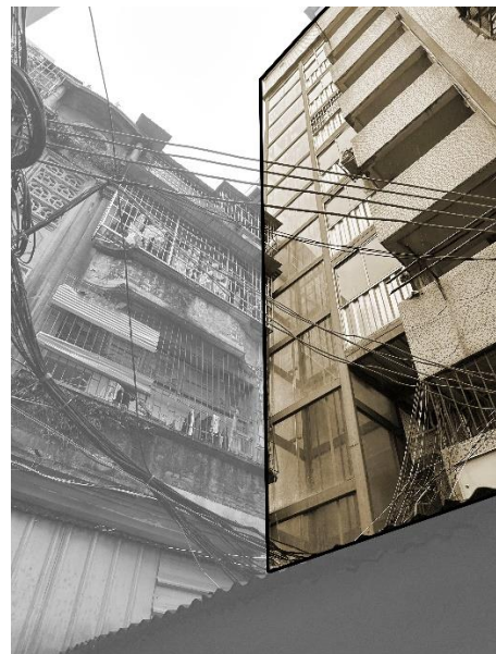
Fig. 5-9 Mosaic tiling, additional hanging ladders (Source: by the author)
