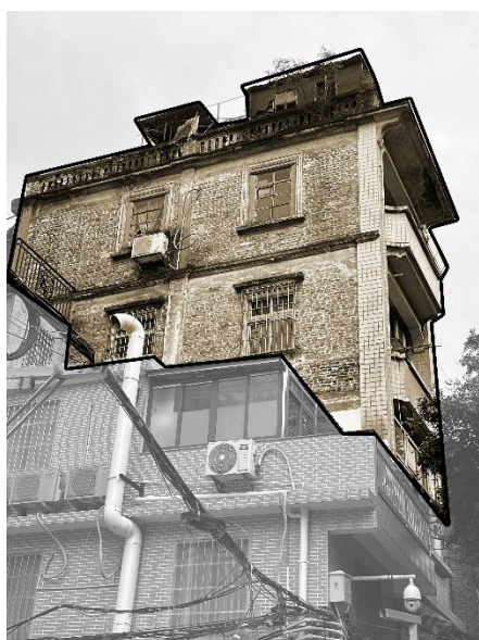
Fig. 5-6 Partial addition of balconies on the roof and brickwork on the facade (Source: by the author)
