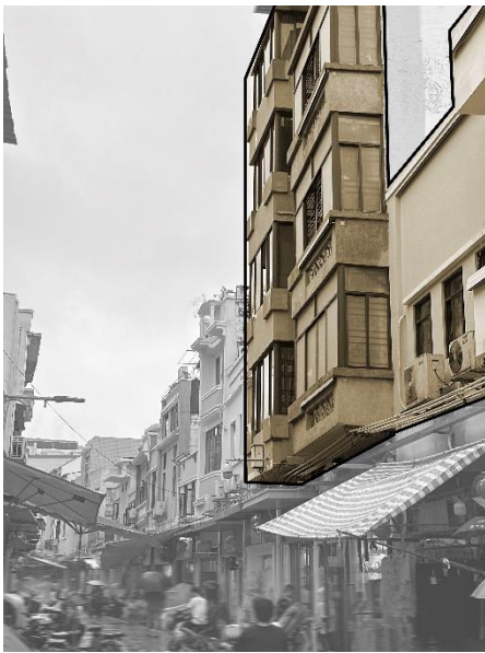
Fig. 5-8 Painted walls and elevations with balcony additions (Source: by the author)
