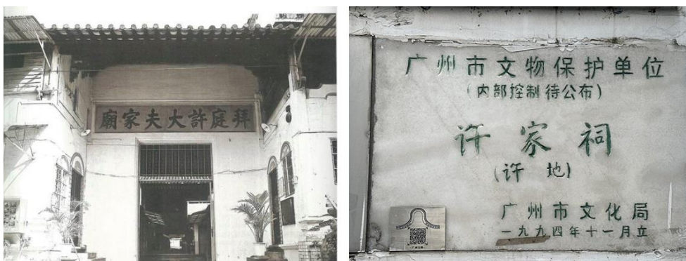
Fig. 4-20 Photos of the Xudi family temple before restoration
