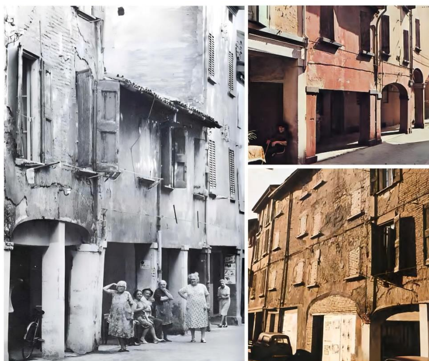
Fig. 2-12 Architectural degradation of the urban area of Bologna (Source: reference [44] )
