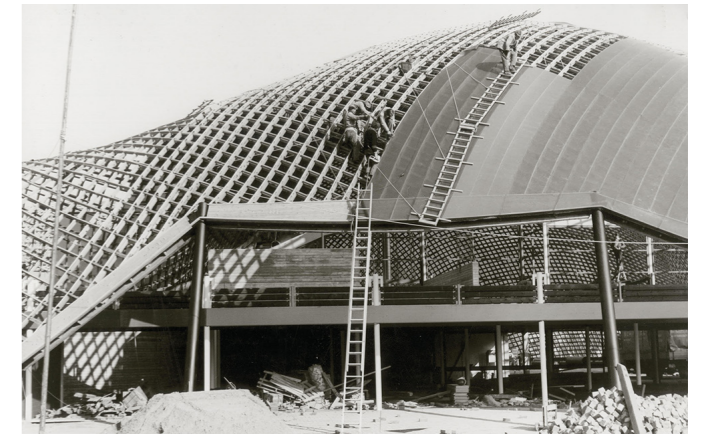
Figure 2.10: Building process of Frei Otto's Mannheim bending-inactive gridshell
