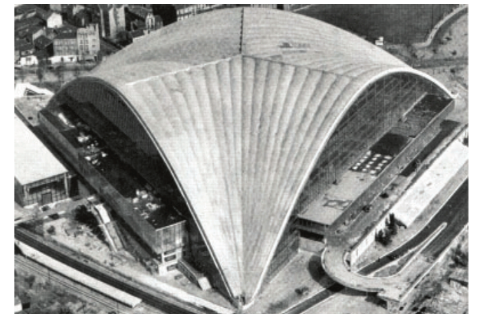
Figure 1.1: Examples of steel-concrete shells
