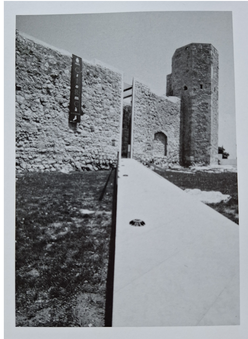
Fig. 3.43. View towards the entrance after the intervention.
