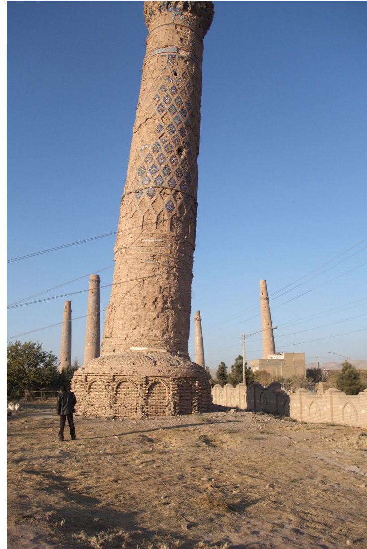
Fig. 1.32. Photograph of the tilted fifth minaret of Herat.
