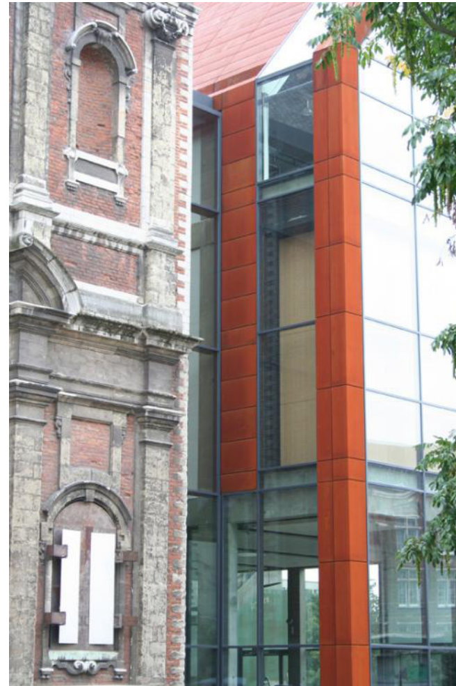
Fig. 3.24. External view of the new corten-clad body connecting to the original chapel (facade detail).
