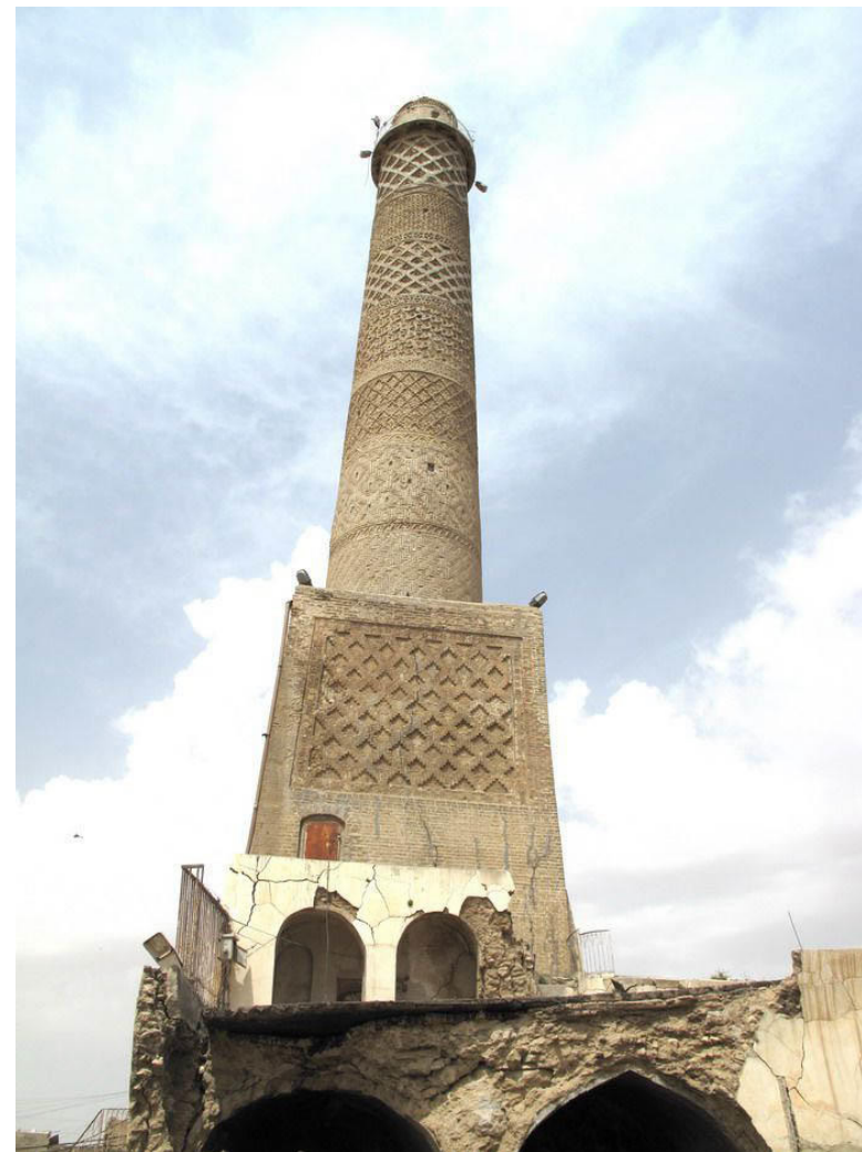
Fig. 1.33. Base and shaft of the tilted Al-Hadba Minaret, Mosul, Iraq, to the internal body of which Bruno and his team had inserted reinforcing micropoles.
