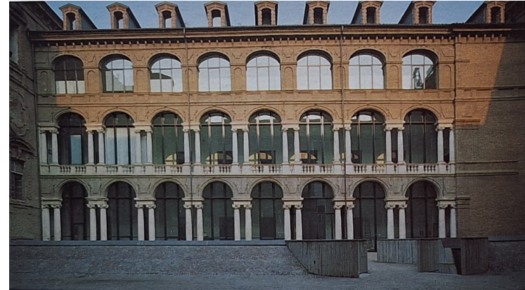
Fig. 3.11. The newly restored facade with the entrance hall from the inner courtyard seen from outside.
