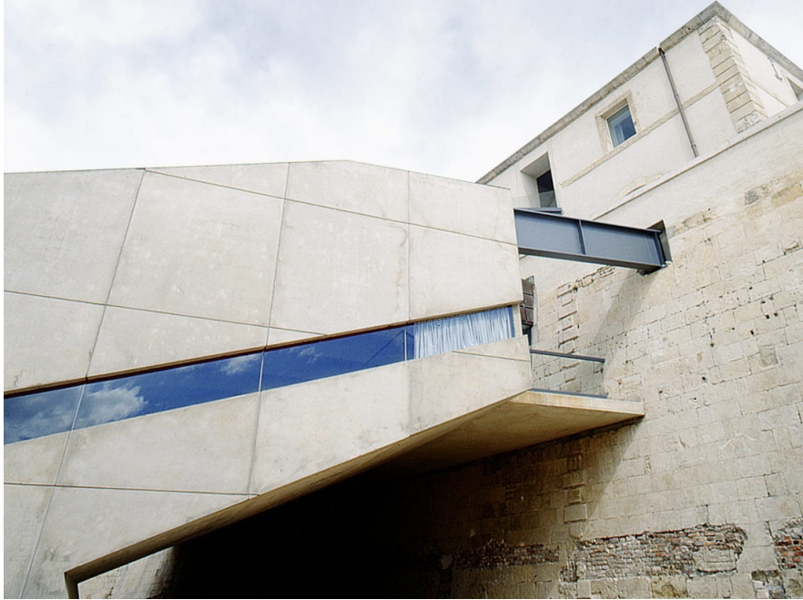
Fig. 3.55. External view of the new amphitheater-classroom. Source: Arch. Ugo Bruno, Cabinet Andrea Bruno. https://www.ugobrunoarchitetto.it/progetto/fort-vauban/
