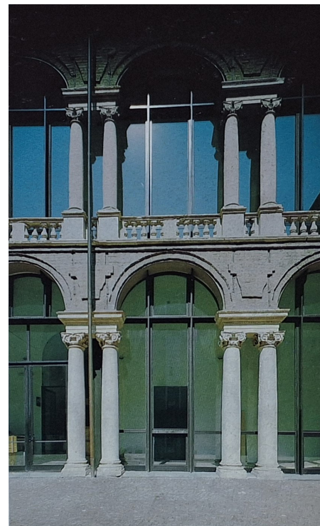
Fig. 3.10. The “window/centering” structure used to consolidate and liberate the original facade.
