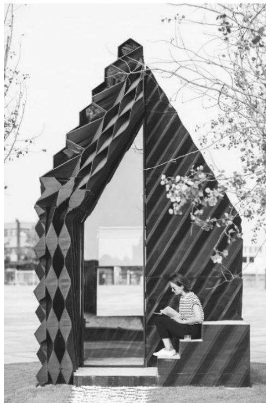
Image 5 The Canal House in Amsterdam, The World's First 3D Printed Canal House Source: (Renner, s.d.)
