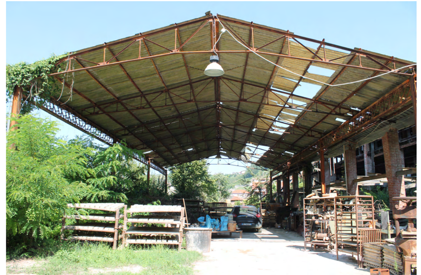
Image 53 Auxiliar metallic structure Source: Photo by the authors, 2024
