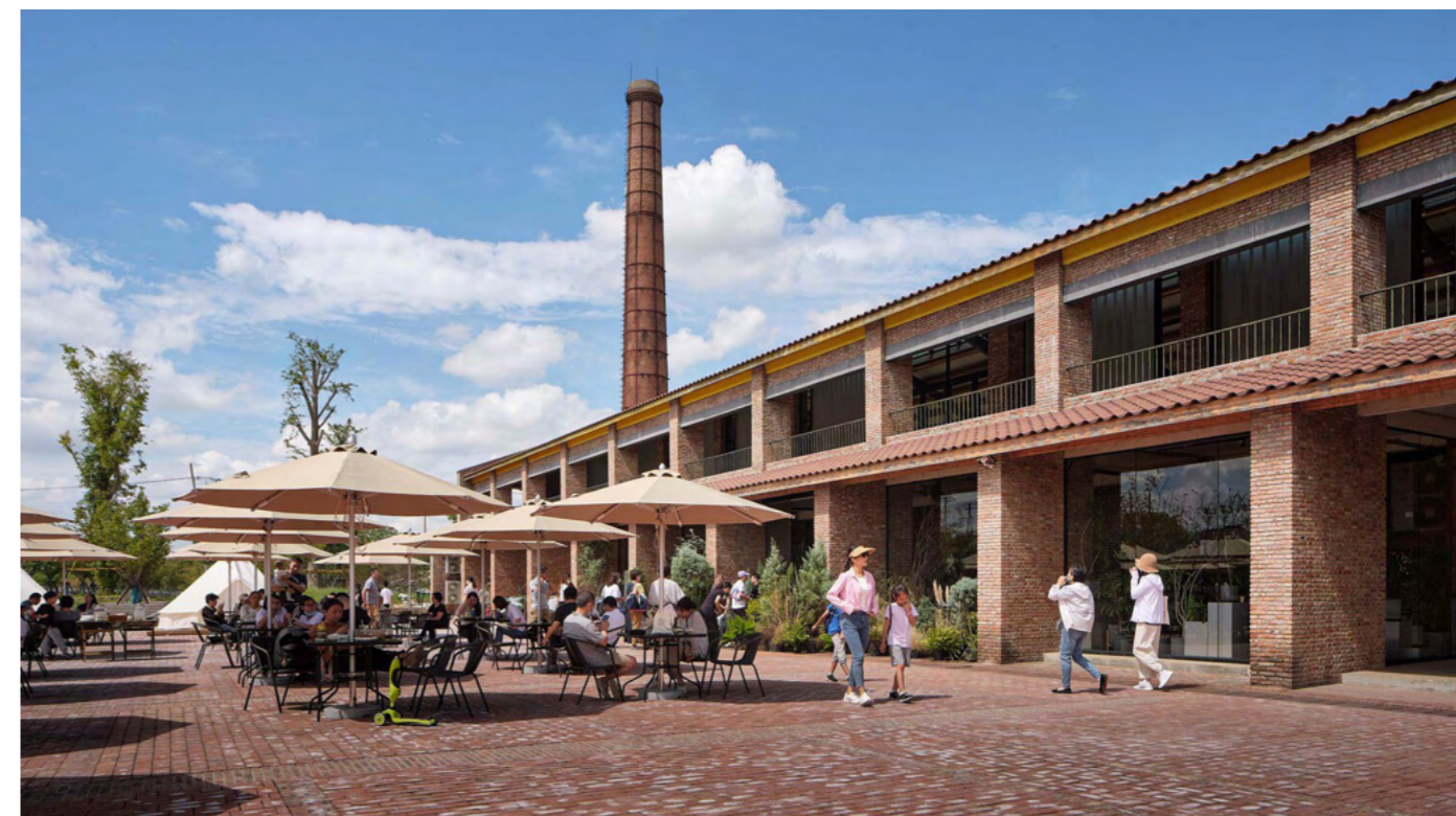
Image 111 Pudong Hoffman Brick kiln renovation Source: Photo by Qingyan Zhu, 2021
