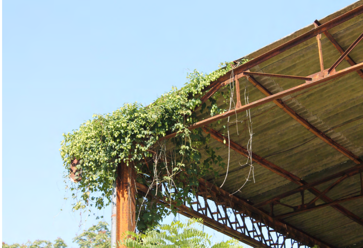
Image 77 Ivy leaved embedded in structure and creating more weight and more moisture Source: Photo by the authors, 2024
