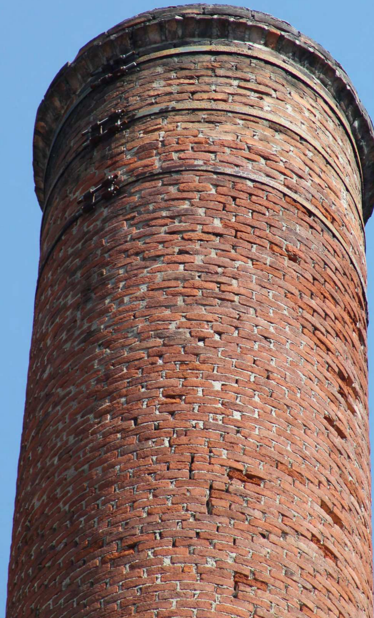
Image 60 Chimney of Hoffmann Kiln Source: Photo by the authors, 2024
