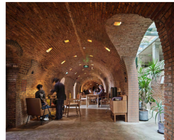
Image 109 Pudong Hoffman Brick kiln renovation Source: Photo by Qingyan Zhu, 2021
