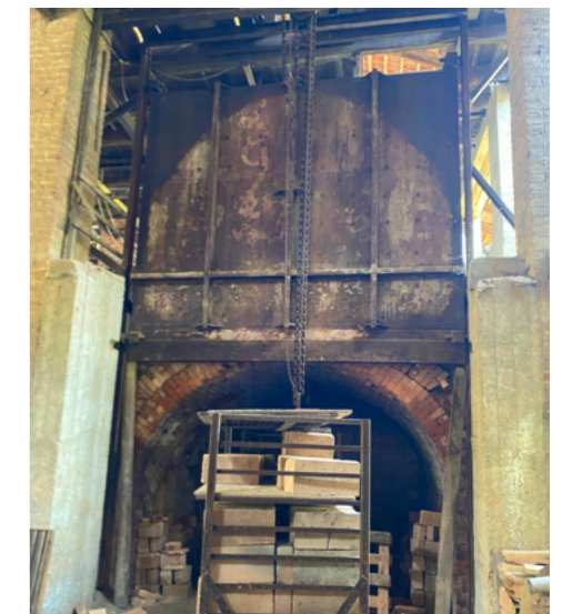
Image 49 Hoffmann kiln doors Source: Photo by the authors, 2024
