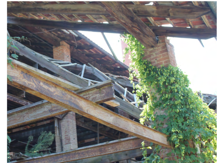
Image 79 Ivy leaved embedded in structure and creating more weight and more moisture Source: Photo by the authors, 2024
