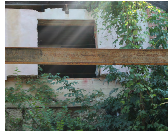
Image 78 Ivy leaved embedded in structure and creating more weight and more moisture Source: Photo by the authors, 2024
