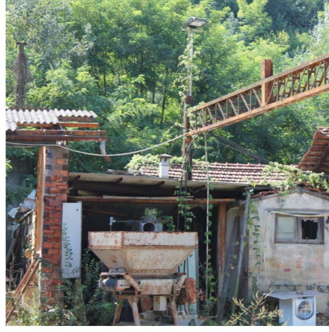
Image 58 Back side of the Fornace Source: Photo by the authors, 2024
