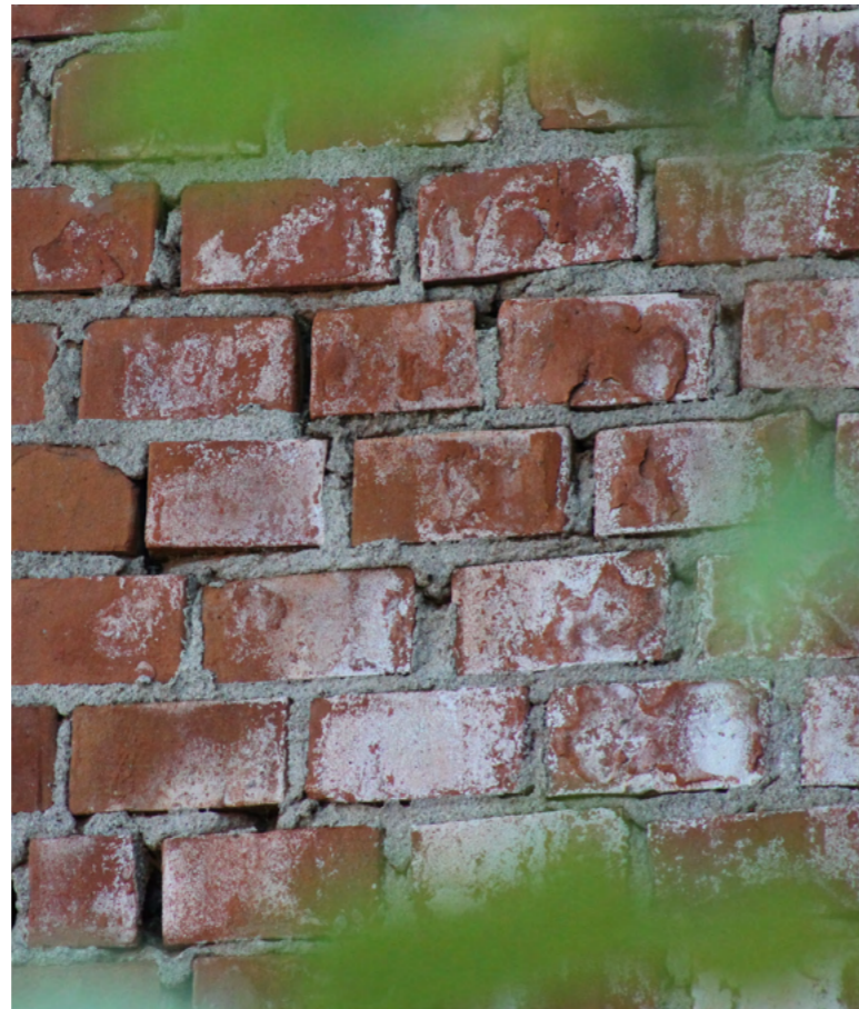
Image 68 Cracks on the Hoffmann Kiln walls Source: Photo by the authors, 2024
