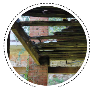
Ref. Image 70 Wood floor, metal beams and brick column
