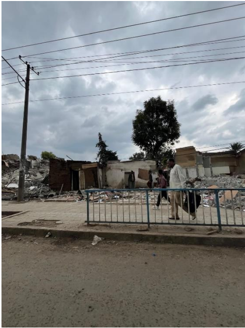
Figure 7-Demolition of neighbourhoods for the new urban project-Addis Ababa 2024-Camilla Paris
