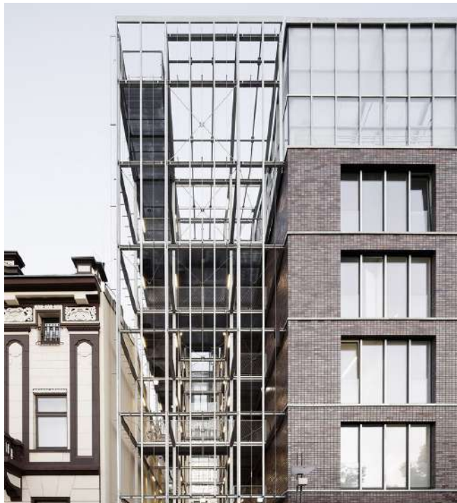
Fig.46 Eastern view of the vertical garden Source: https://kuehnmalvezzi.com/
