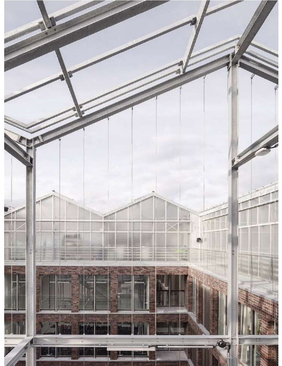
Fig.48 Viewing the courtyard from the rooftop greenhouse
