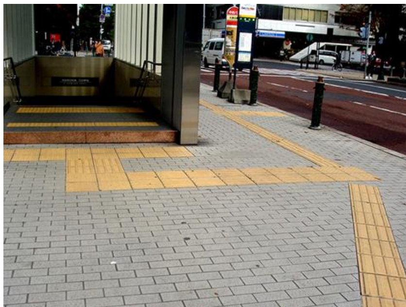
Figure 83: Meanings of Tactile Paving: A Blessing for Persons with Visual Impairment. (Lalit, S. ,2018, March 18).
