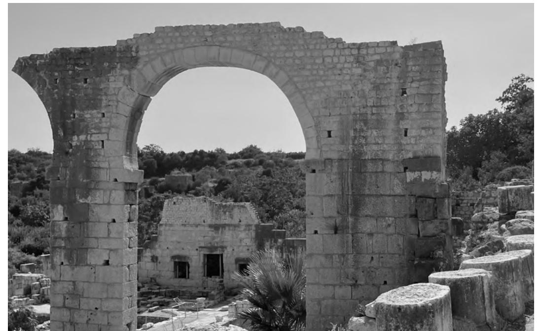
Figure 20: After restoration works
