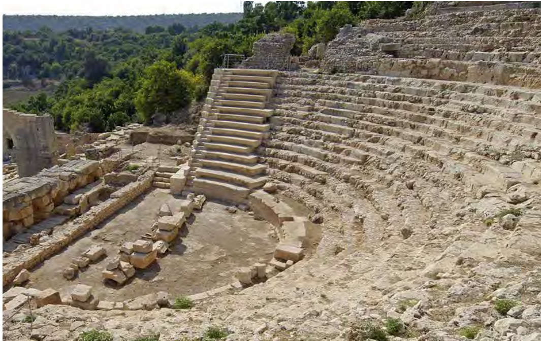
Figure 21 The Restored portion of the theatre
