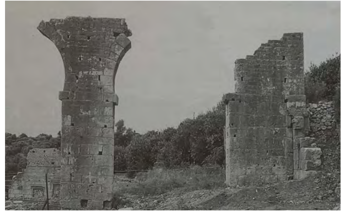
Figure 19: Before restoration works
