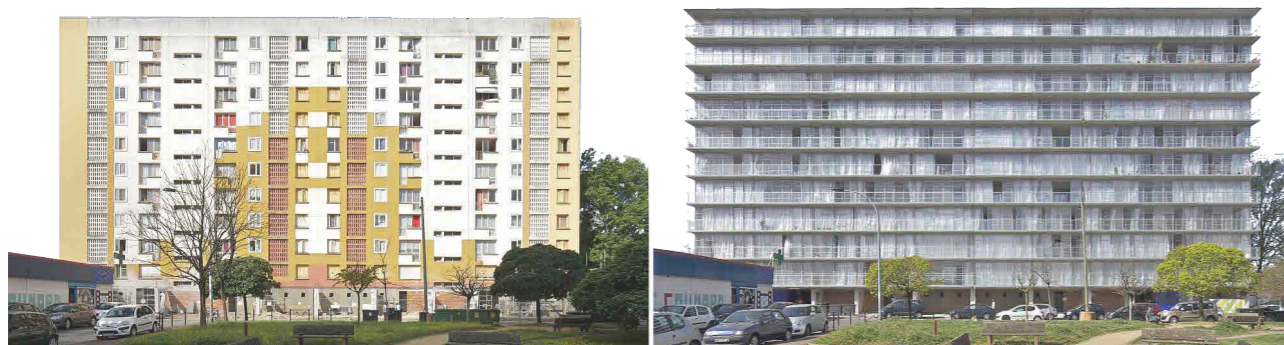
Figure 2.1: Previous condition of the façade & after the new space extension (1)
