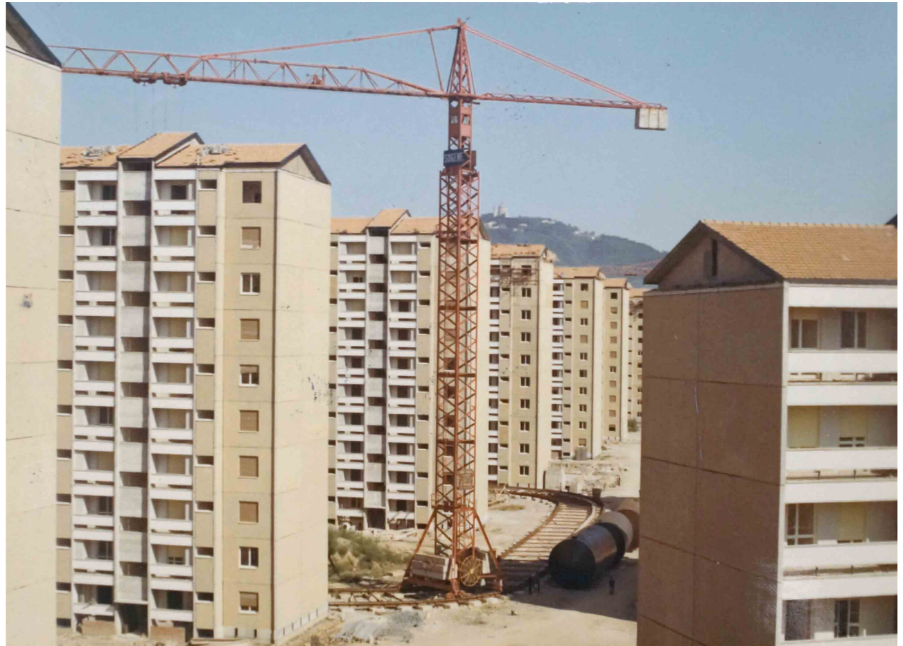
Photo showing installation and construction process, taken from ATC archive.
