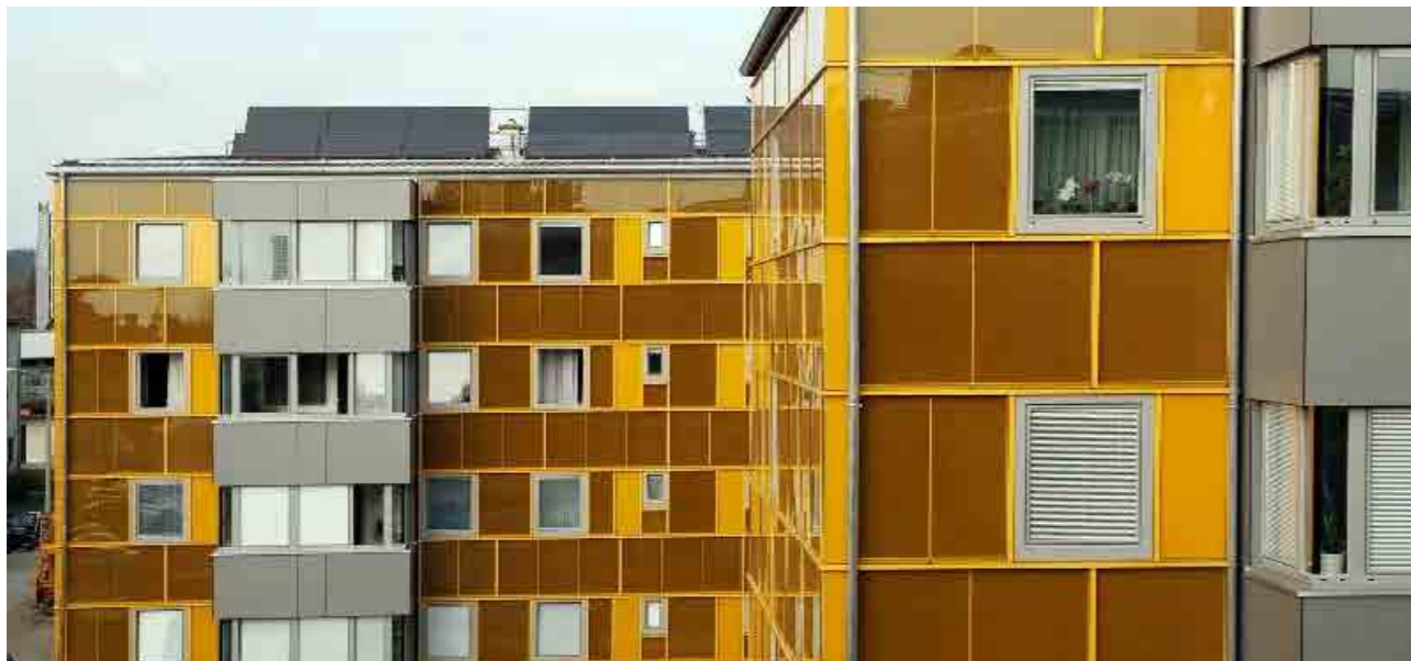
Figure 2.31: Trombe wall façade renovation (17)
