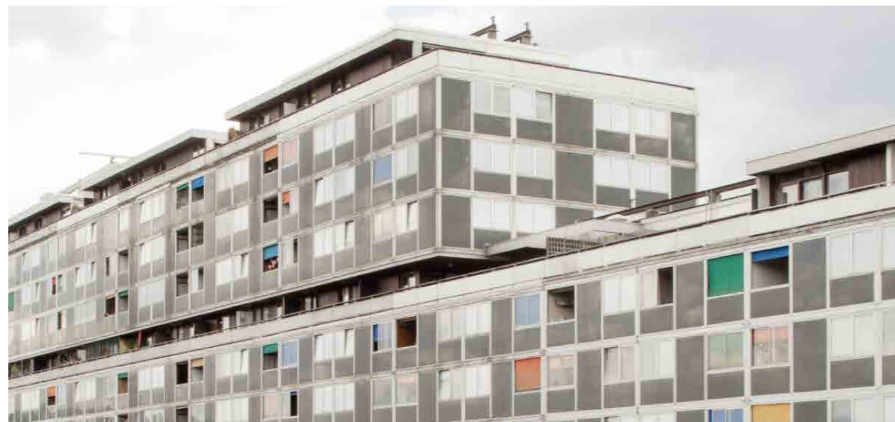
Figure 2.10: Retrofitted façade of the Du Lignon (7)
