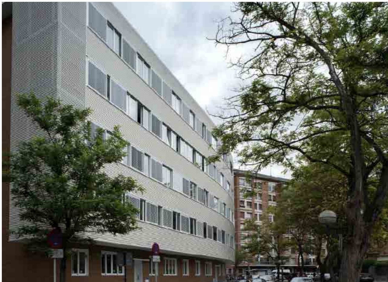
Figure 2.38: Coverage of the existing balconies designed to show as one mass (23)
