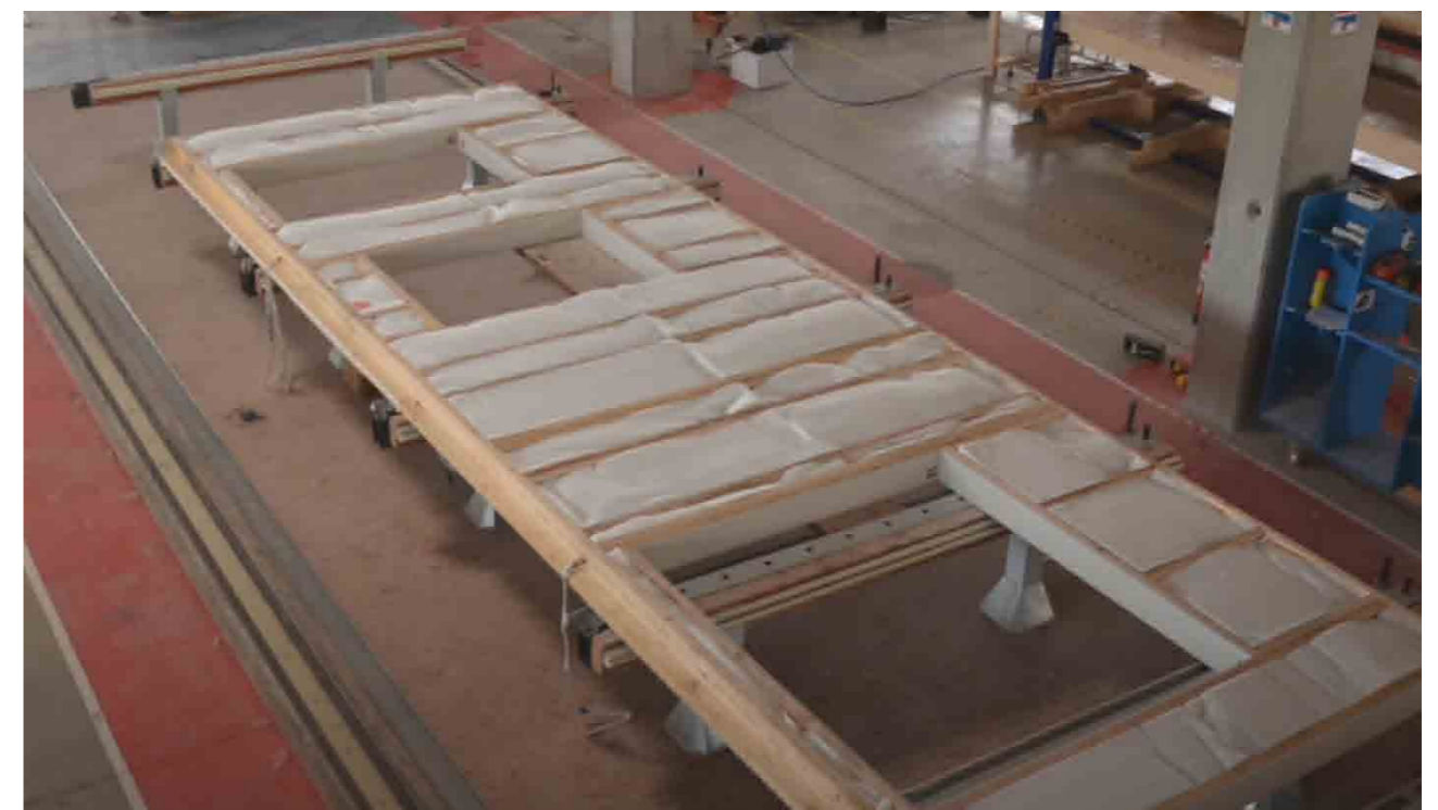
Figure 2.37: Construction process screenshot taken from the refurbishment video (22)
