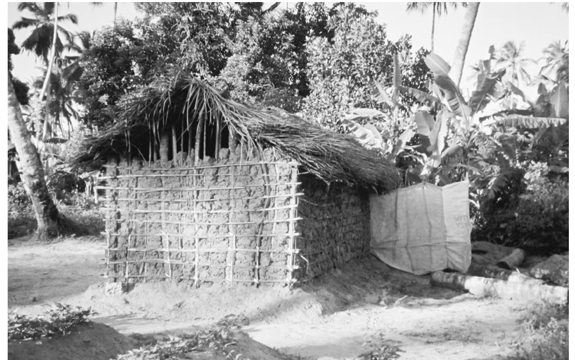
Picture 4.3. Fito frame with udongo (mud) walls, Mwera, Zanzibar. (Photo by Garth Myers, 2006)
