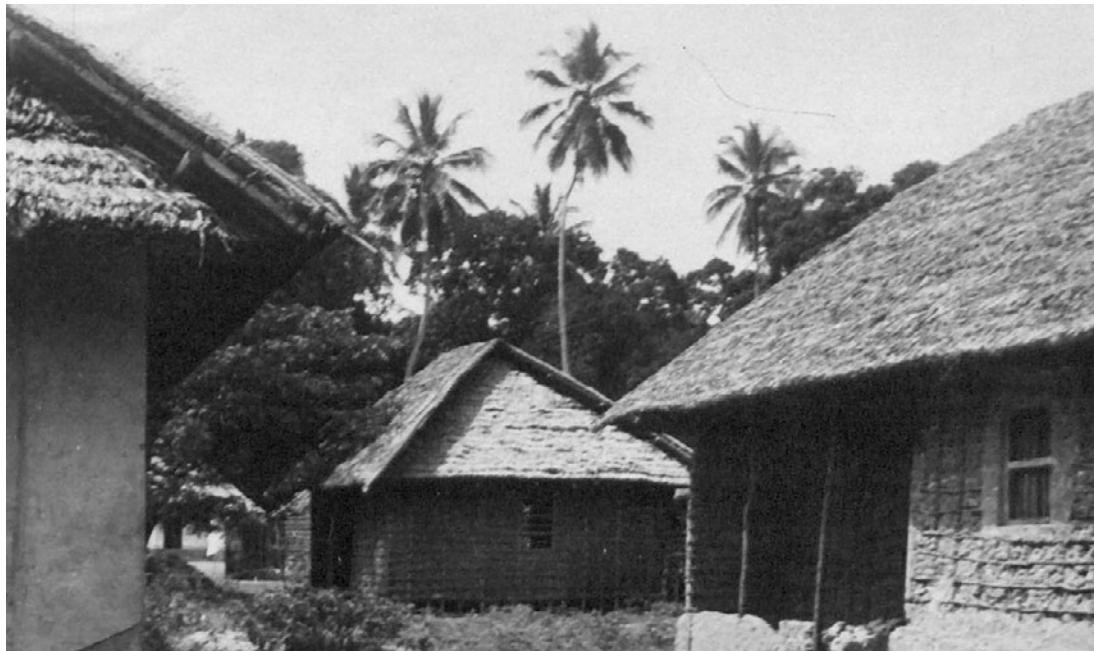
Picture 4.2. Native huts, showing boriti and fito (pole and lath) walls filled with mud or lime mortar and topped by makuti (thatch) roofs, Ng'ambo area, Zanzibar. (Photo by Henry Pilling, 1944)
