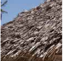
Straw/dry leaves Wooden rafters
