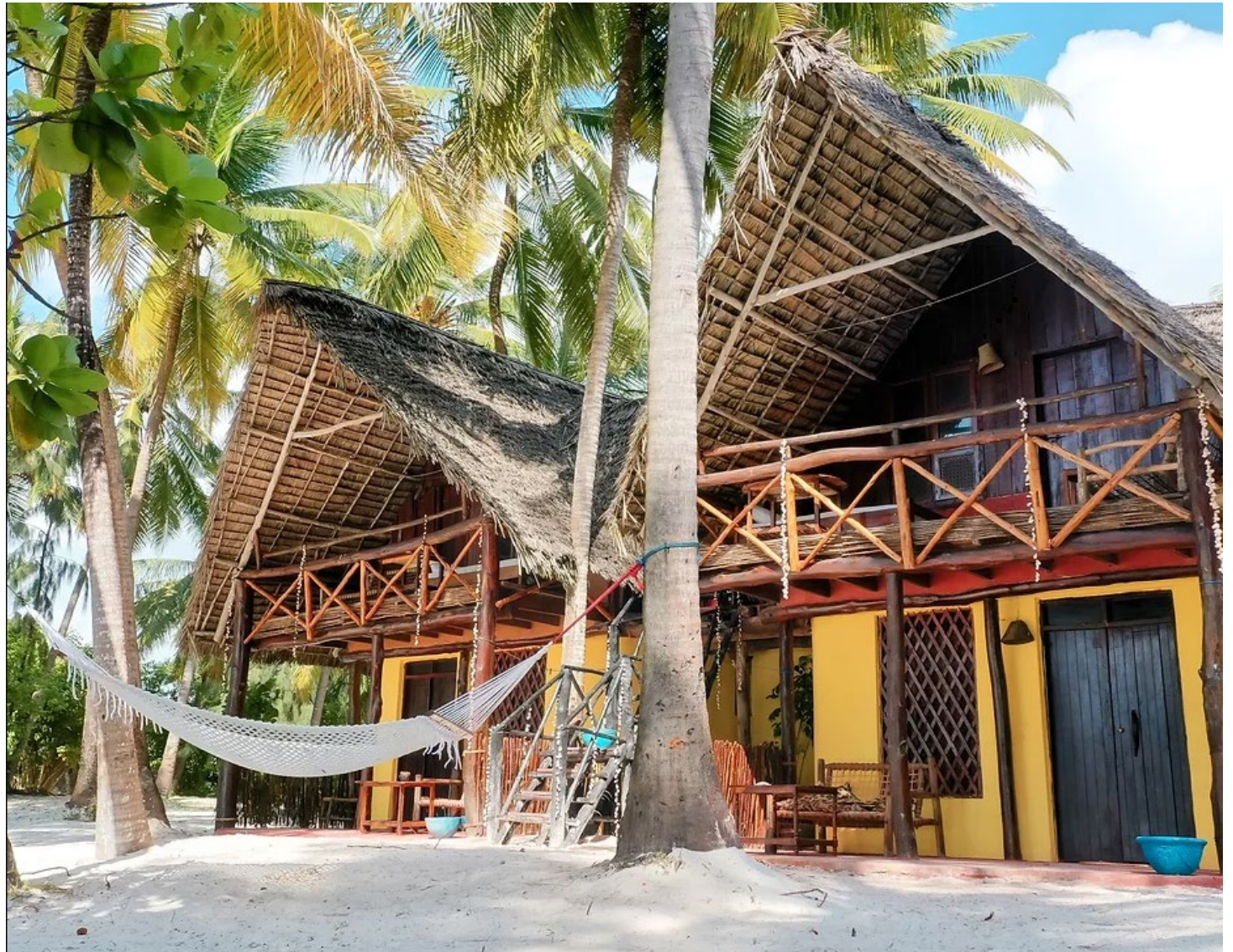
Picture 3.12. Two story double residential units of the Evergreen Bungalows resort. (Image source: Evergreen Bungalows website. Accessed November 24, 2024)
