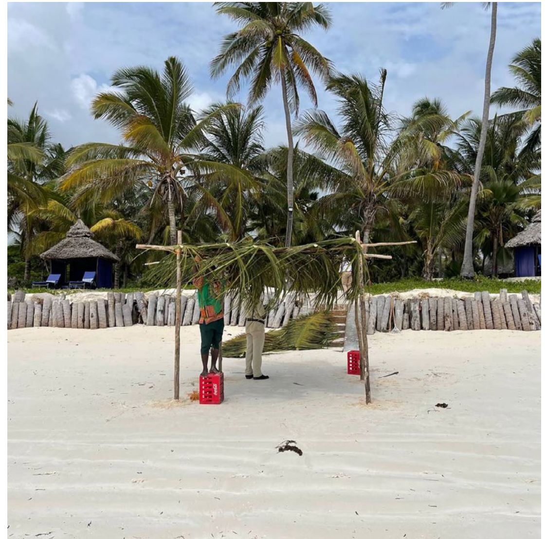
Picture 1.4. Local workers assembling temporary structures using coconut palm leaves. East coast. Territory of Breezes Beach Resort (photo by author, february 2021)
