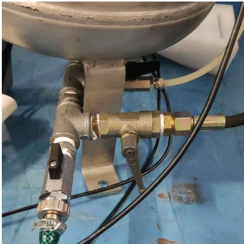
Figure 30: Valves installed at the base.
