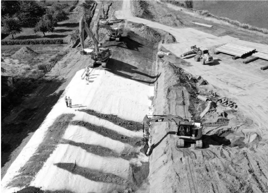
Figure 1.11 Application example of bentonite geosynthetics - source: 'Geosynthetics and sustainability GEO kunst special 2022'.
