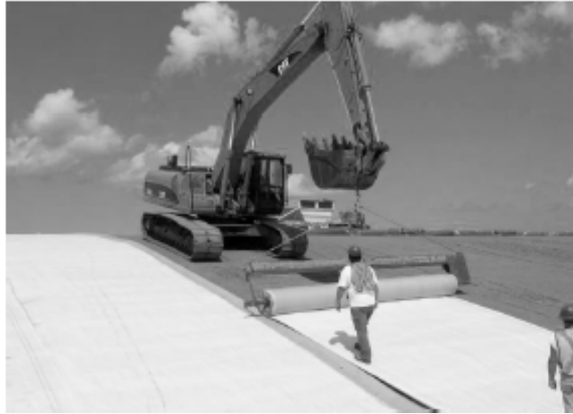
Figure 3.14 GCL Installation phase - Source 3-K-VON-MAUBEUGE-Naue
