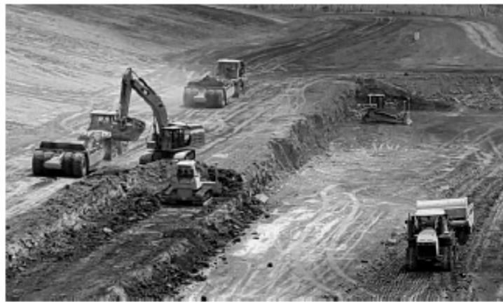
Figure 3.13 Subgrade preparation and clay spreading - Source 3-K-VON-MAUBEUGE-
