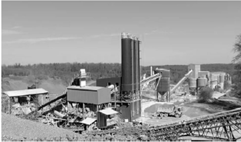
Figure 3.6 Processing of Clay - Source 3-K-VON-MAUBEUGE-Naue
