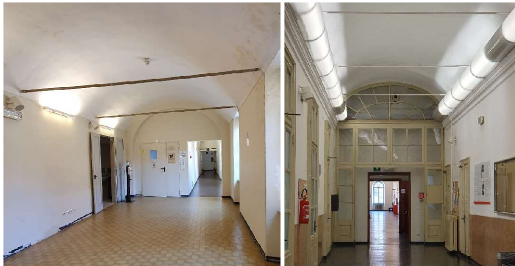
Figure 5.31. Halls of Palazzo Campana, showing vaulted slabs with metal tendons
