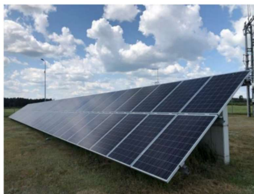
Figure 3-1 - Experimental setup consisting of the pc-Si PV modules under study[34].
