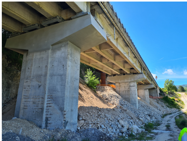
Figure 4.2: View of the Le Pastena bridge.
