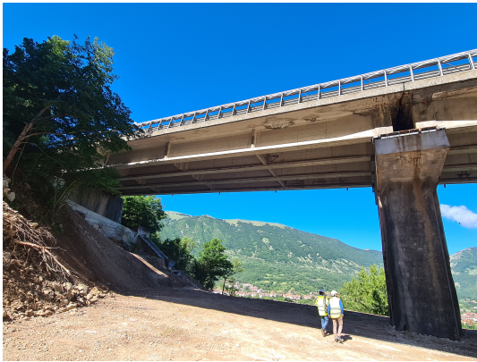
(a) General view of the left span of the Cerqueta bridge.
