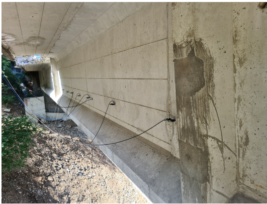
(a) Left span of the Cerqueta bridge.
