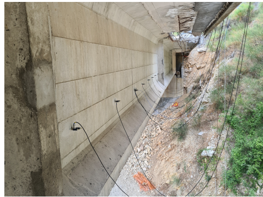
(b) Right span of the Cerqueta bridge.
