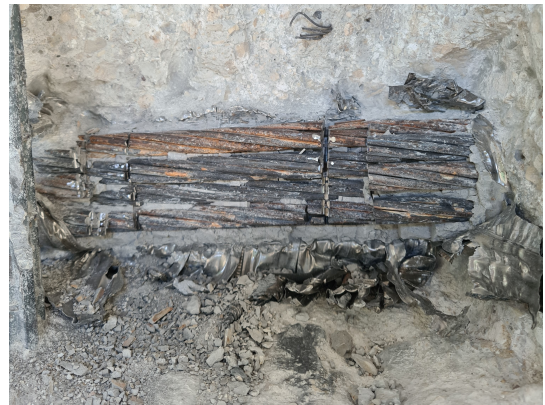
(d) Close-up of cable arrangement after cut on Cerqueta Bridge.
