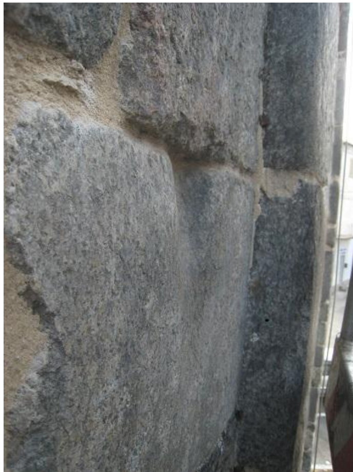
Detail of a bell tower
