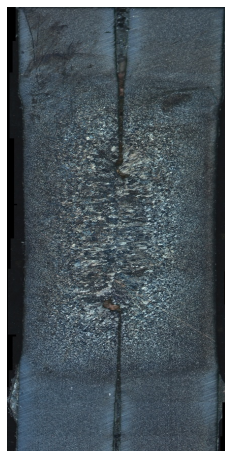
Figure 3.5: The Detail of a weld
