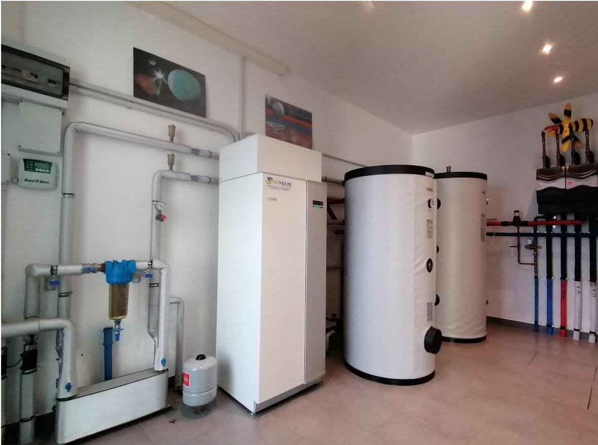
*Figure 35 Heat pump NIBE F12345 and buffer tank*
