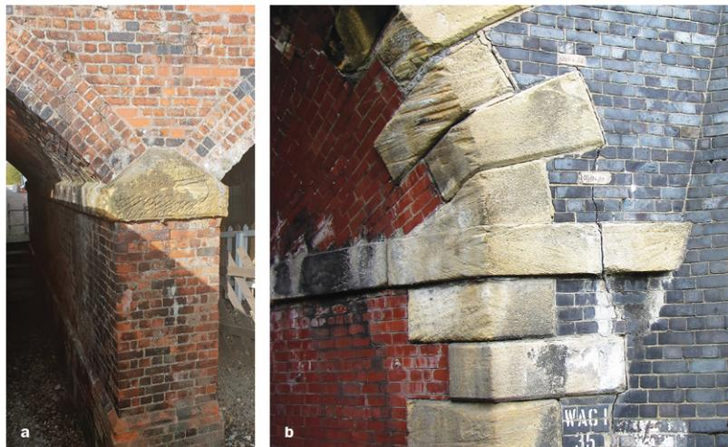
Figure 2.3. Brickwork arch bridges featuring various stone masonry elements: (a) skewback and (b) quoins [12].
