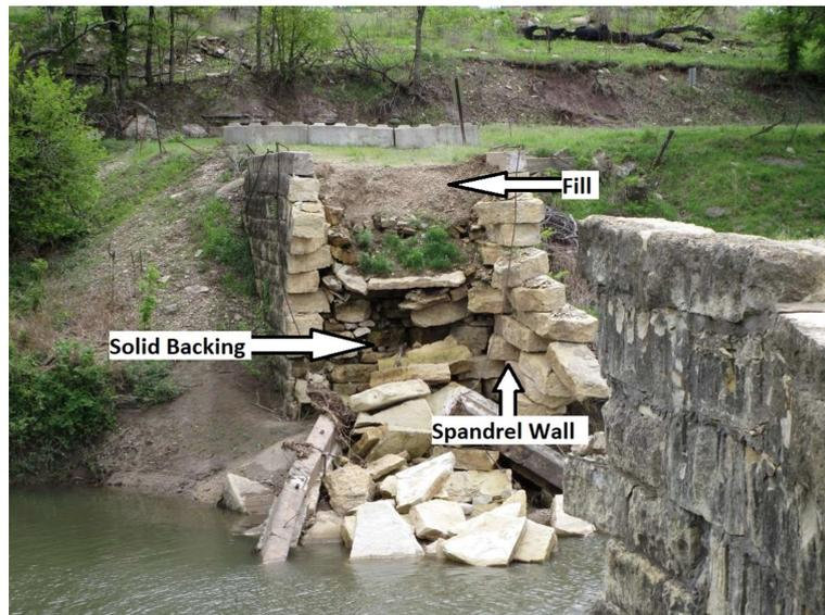
Figure 2.20. Backing and spandrel walls [31].
