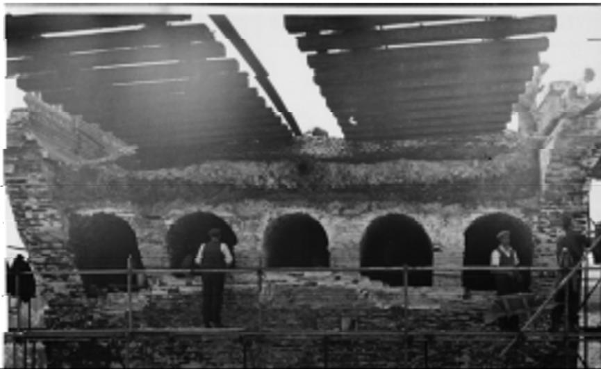
Figure 2.21. Internal spandrel walls [16].
