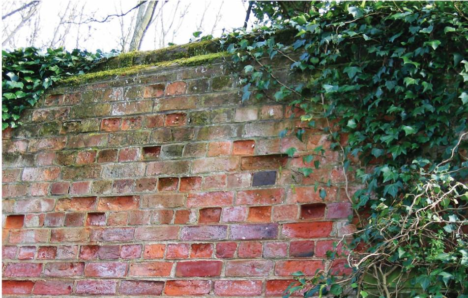
Figure 2.5. Degradation of bridge parapet, likely due to freeze-thaw action [12].
