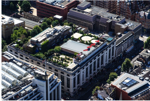
Figure 2.5: Kensington Roof Gardens in 2017
