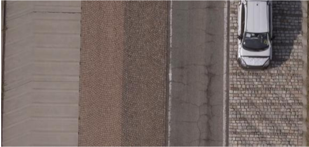
Figure 1 In this picture we can notice from left to right: the short-wave paving, the Procaccini paving, the Swiss Italian pavé, a bumpy asphalt and finally the Belgian cobblestone
