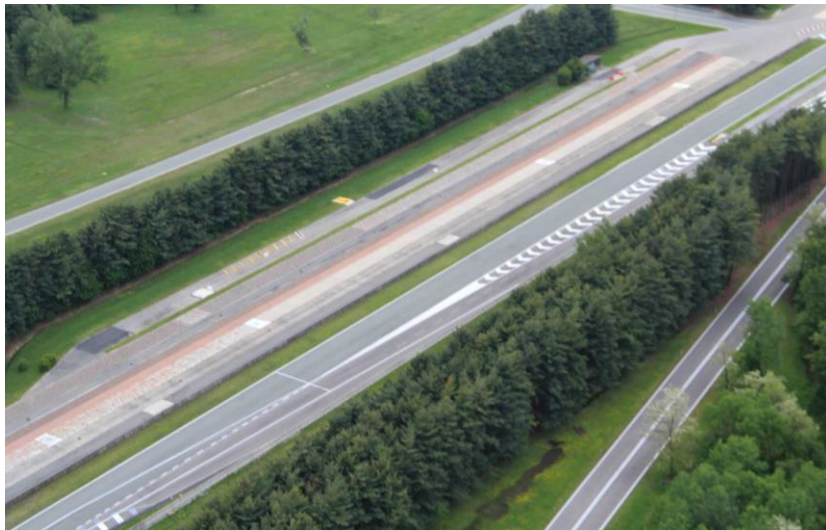
Figure 2 View from above of the Alfa special paving tracks
