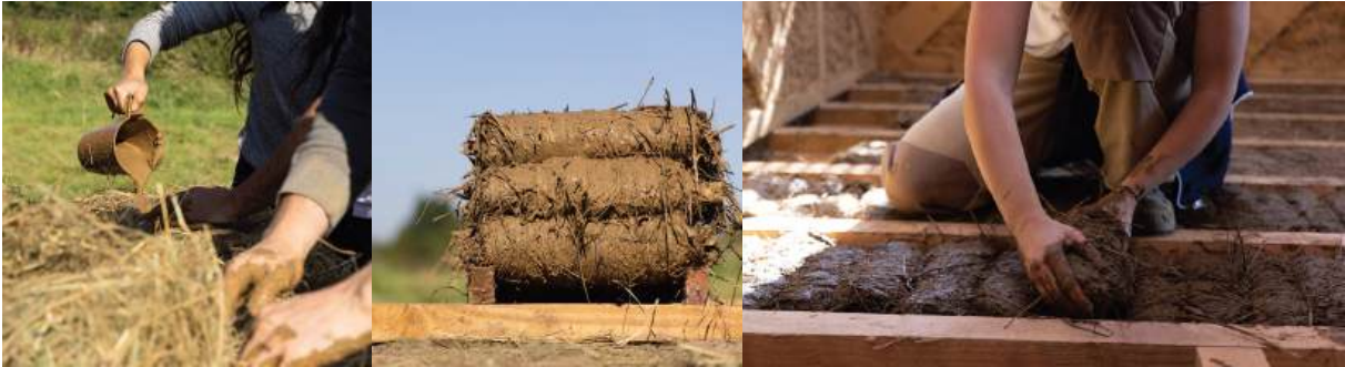
Figure 33. "quenouilles" raw earth, wood sticks, straw and clay Source: Anatomies d'Architecture. (2023, March)
