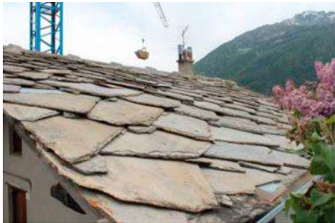
Figure 23. Calcschist CM roofing in Lignod after renovation Source: Journal of Building Engineering
