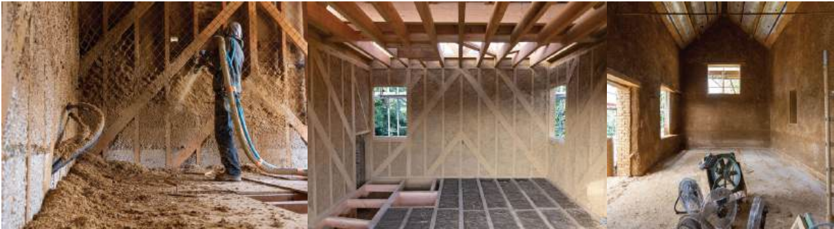
Figure 34. Hemp insulation installation Source: Anatomies d'Architecture. (2023, March)
