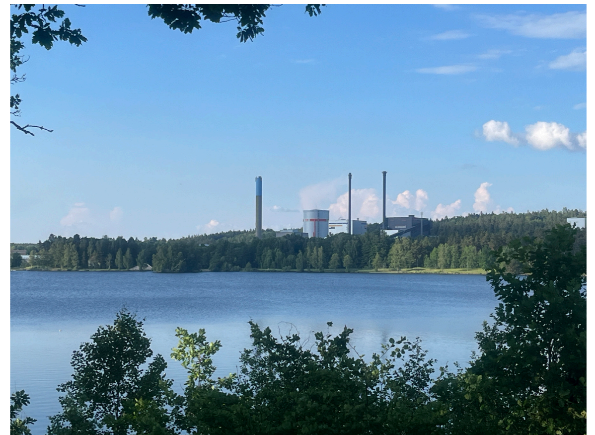
Figure 22: Sandvik thermal and energy plant (Photo by the author 2024)
