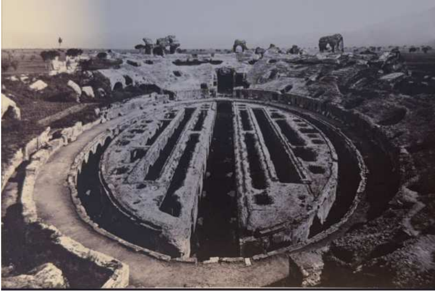
Figure 6 Ruins of the Flavian Amphitheater, Santa Maria Capua Vetere, 2nd century BC. Note the underground passages. Photo © Alinari/New York, 《Art Resource》
